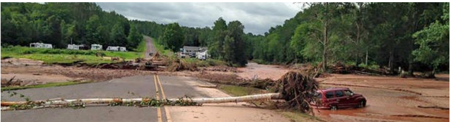
Water breached the stream banks and washed out CTH A at the bridge over Oronto Creek, as well as the campground and marina.
