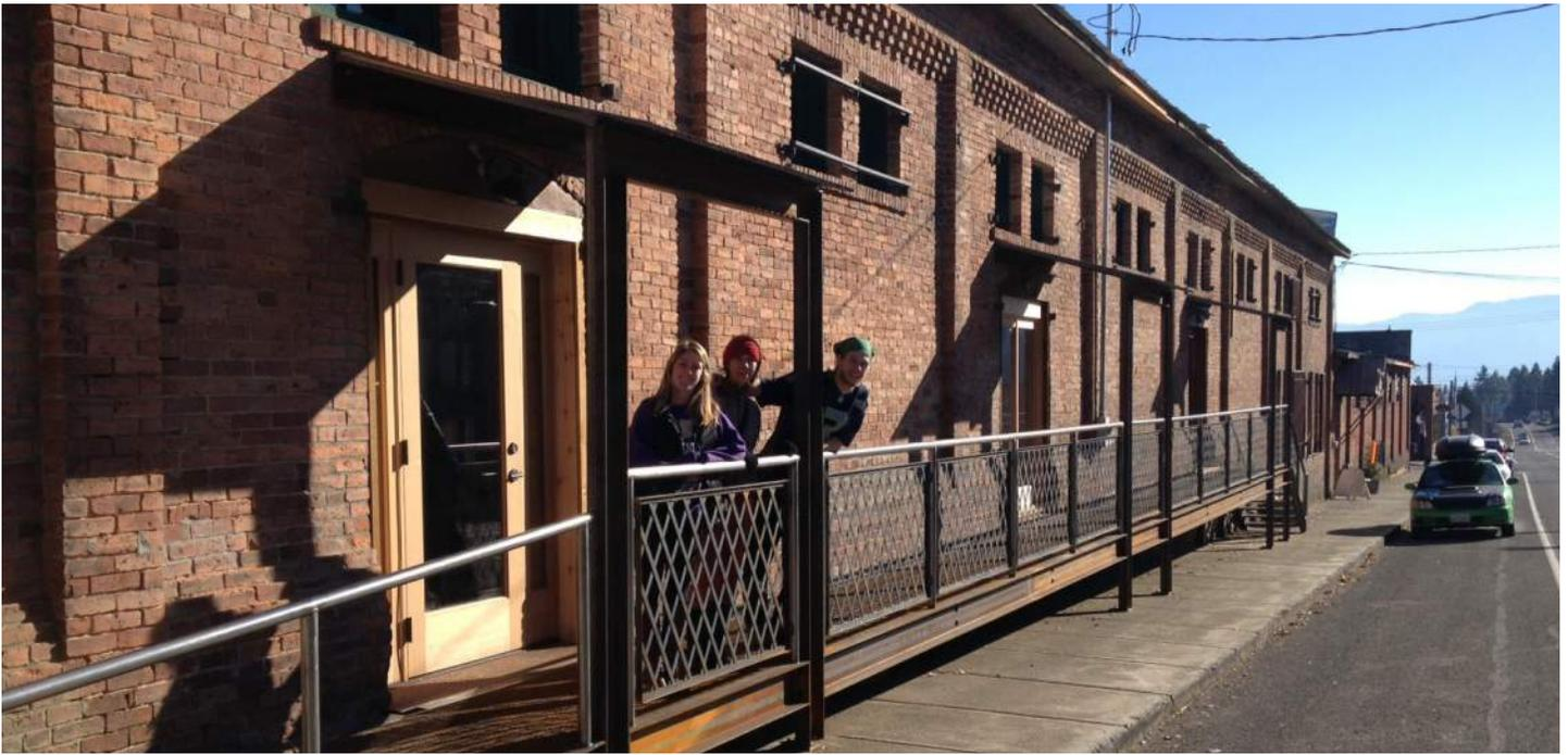
Phase one work included a new ADA compliant ramp, walkway and stair along the west sidewalk providing access to retail and event spaces. Steel-framed canopies protect the entries from rain and snow.
