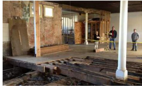
Phase one work included structural repair of the wood floor framing.
