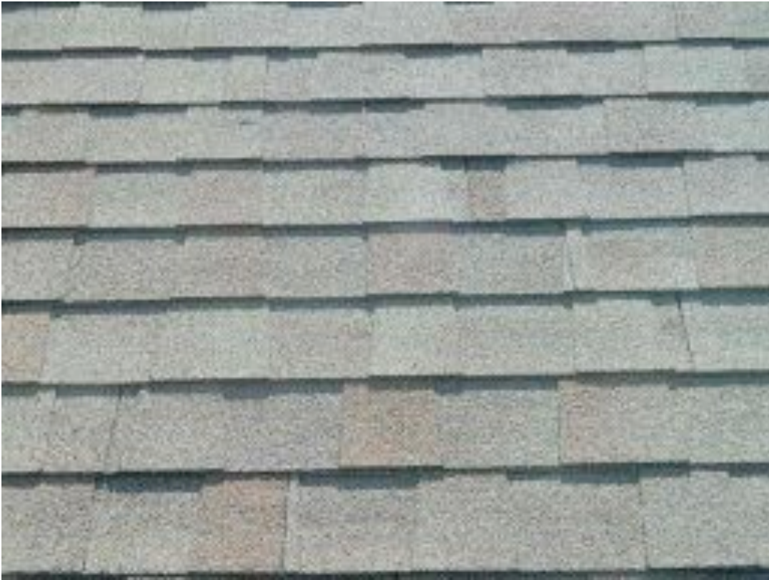
FIBERGLASS-REINFORCED RANDOM TAB SHINGLES
