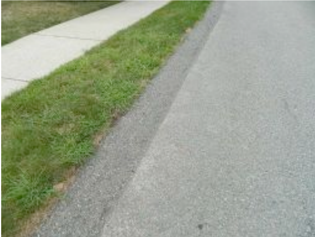
TYPICAL EXTRUDED CAPE COD BERM
