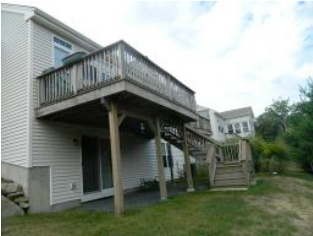
TYPICAL ELEVATED OPEN WOOD DECK
