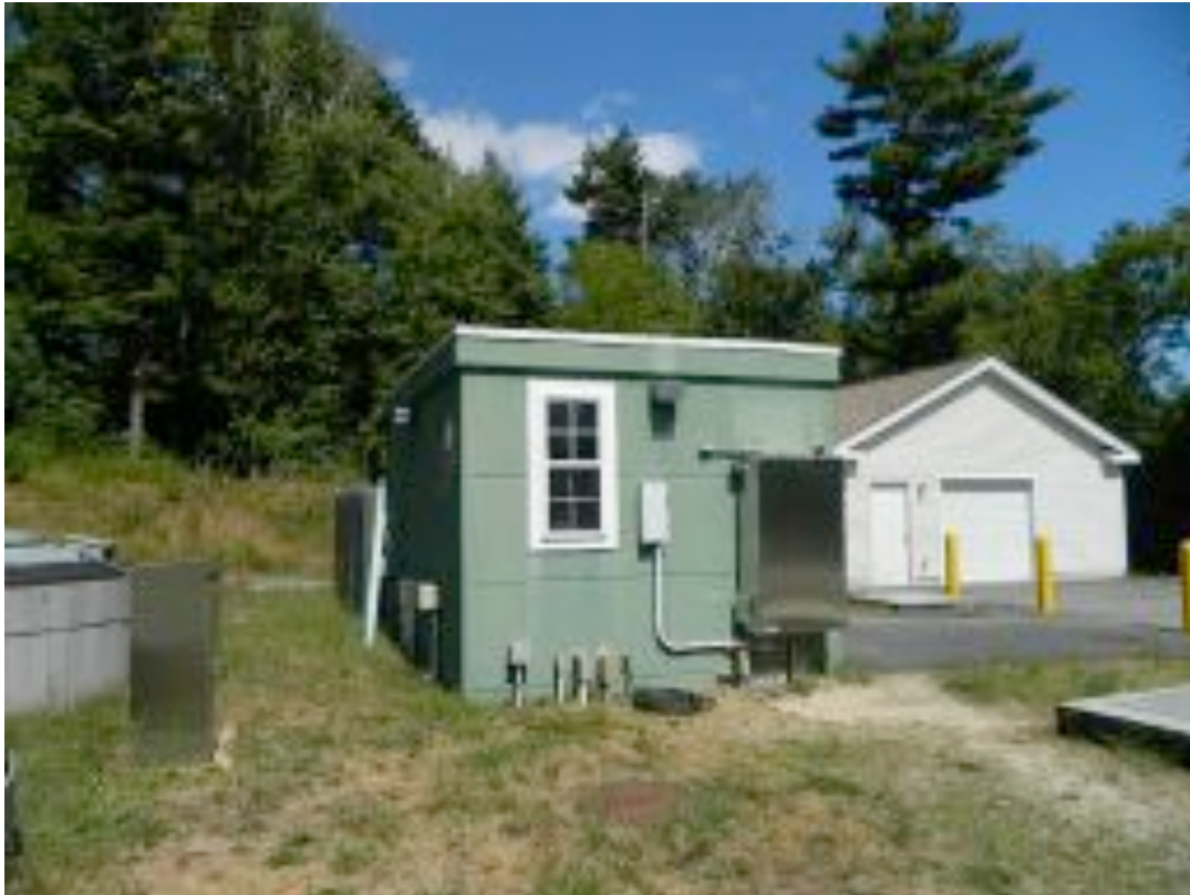
WWTP CONTROL BUILDING
