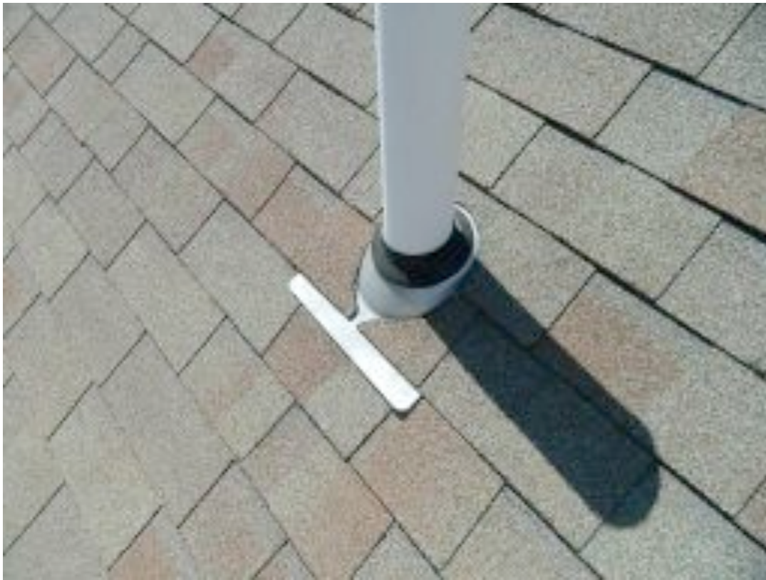
TYPICAL NEOPRENE/ALUMINUM PIPE FLASHING
