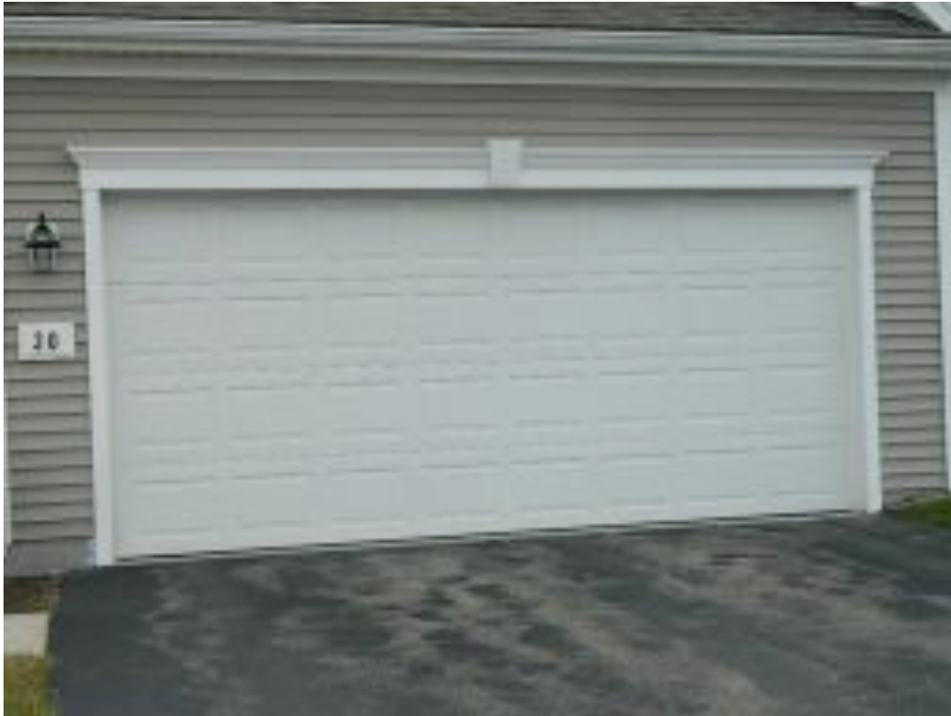
TYPICAL 16 X 7 INSULATED METAL OVERHEAD DOOR
