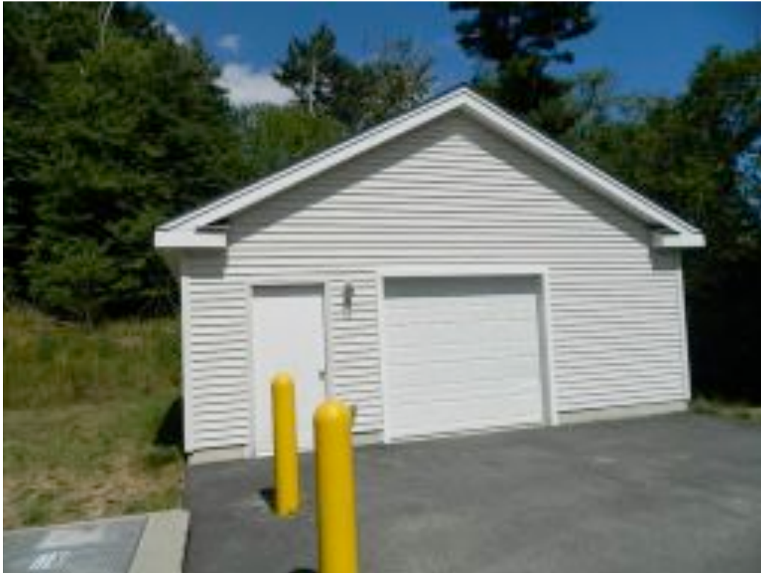
OVERVIEW OF THE WWTP AREA STORAGE GARAGE
