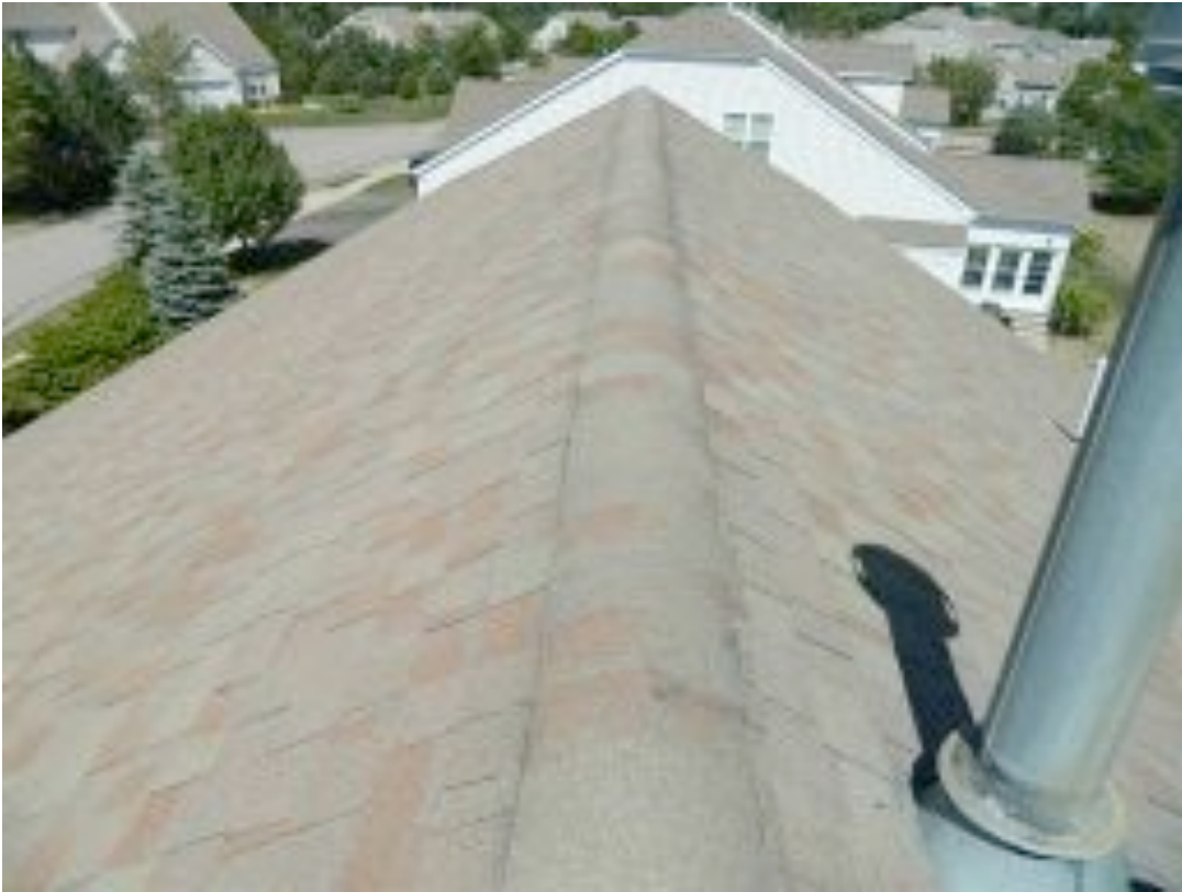
TYPICAL SHINGLED-OVER RIDGE VENT
