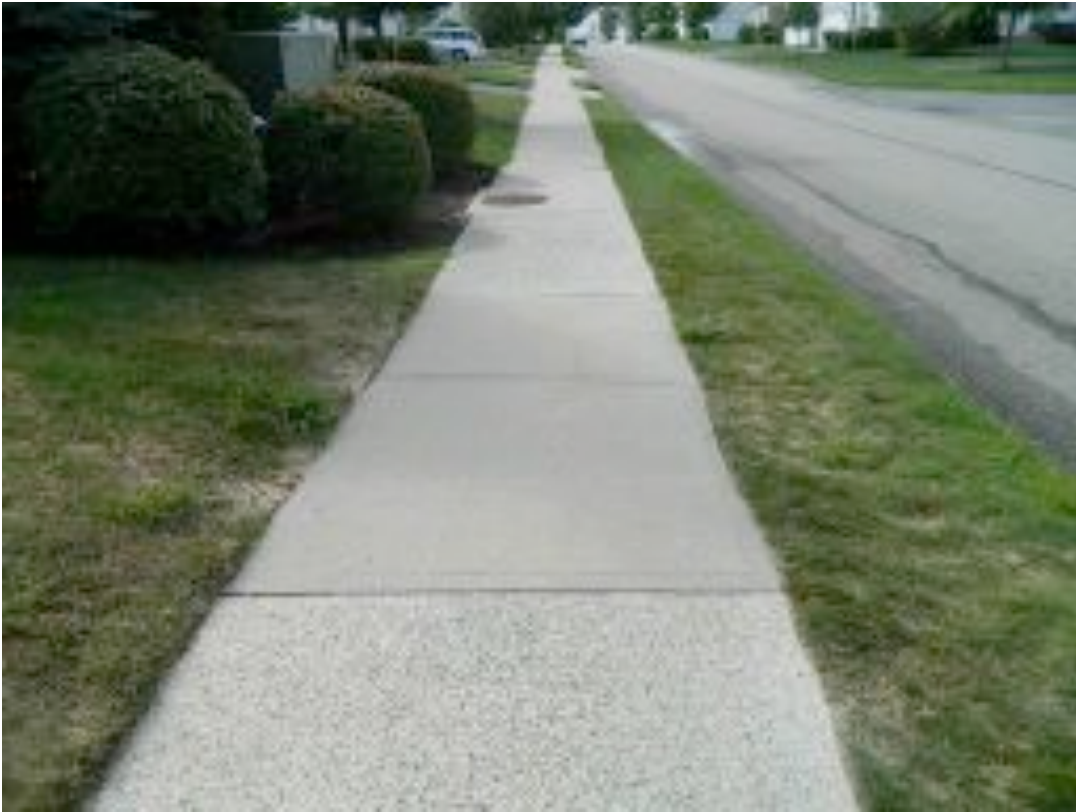
SOME INDIVIDUAL PANELS HAVE BEEN REPLACED
