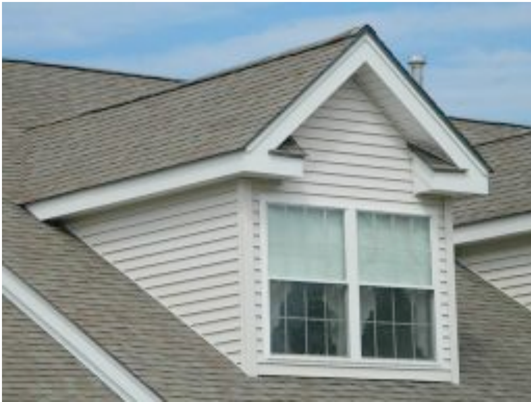
TYPICAL ABOVE-ROOF WINDOW DORMER
