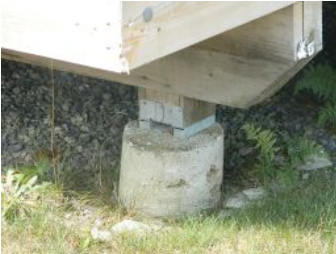
THE DECKS REST ON POURED CONCRETE FOOTINGS
