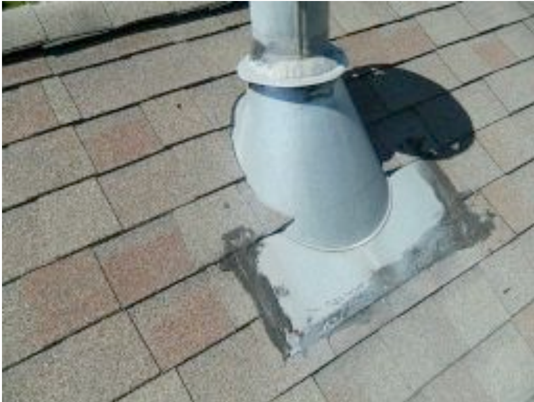
TYPICAL TYPE B GAS VENT STACK FLASHING
