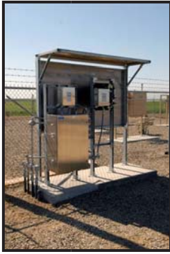
Fig.2 – Field installation of TDLAS
