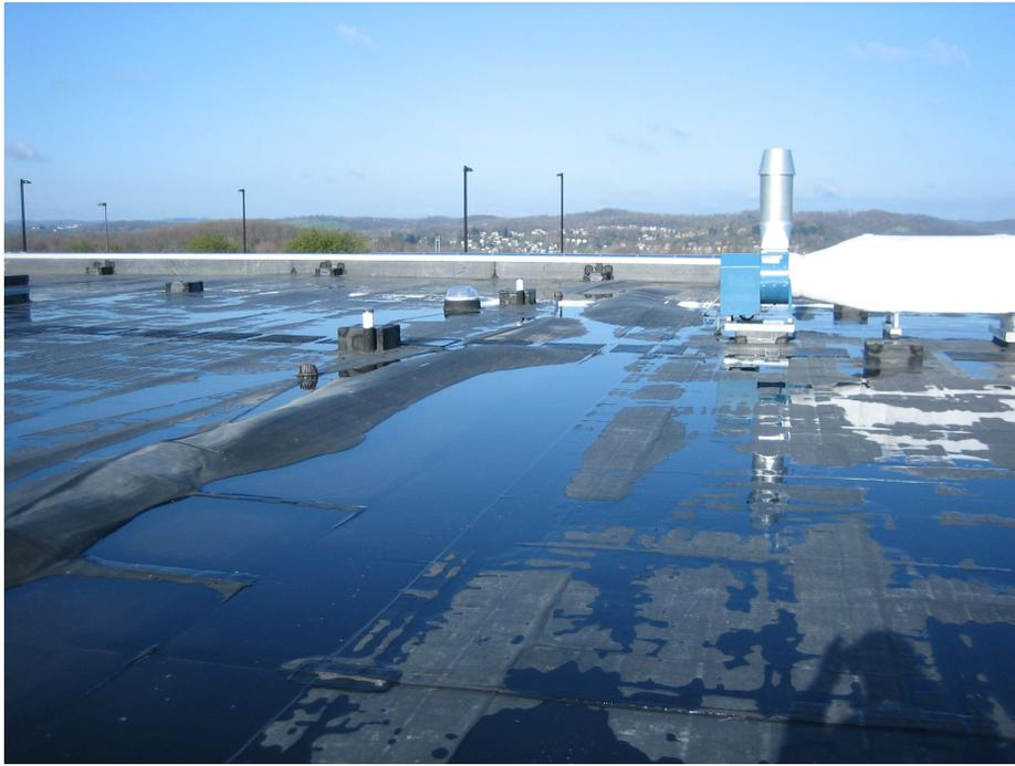
Photo 1 The photo demonstrates the typical condition of a recently installed fully adhered roof system over lightweight structural concrete. Bead adhesives were used to install insulation boards directly to the deck; no cover board was used.
