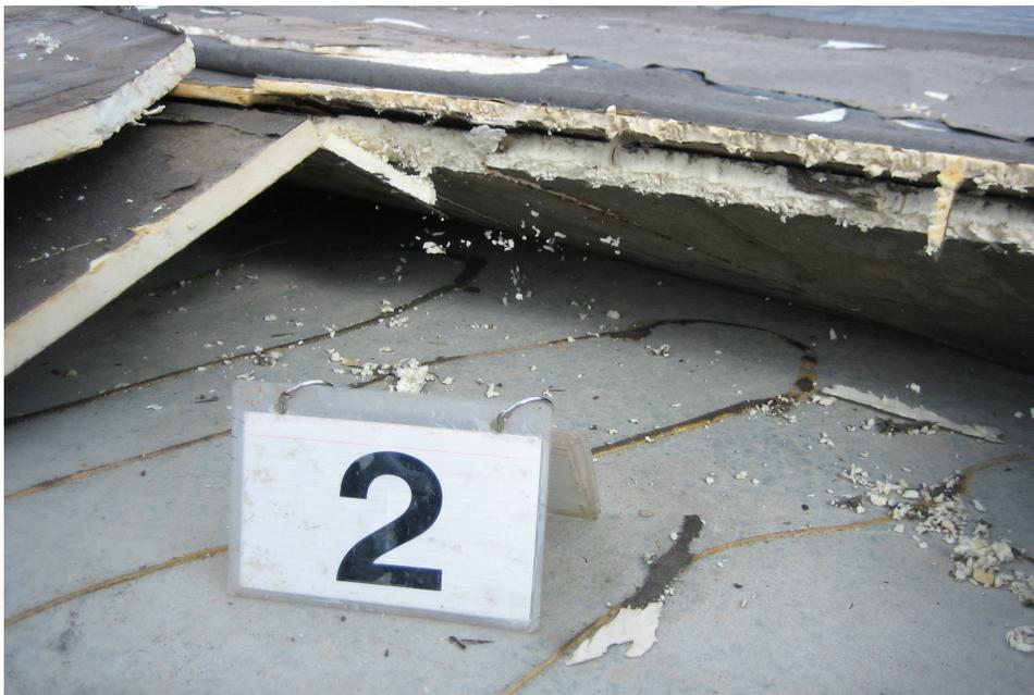
Photo 3 This is another area of the roof described in Photo 1 showing pronounced dimensional stability issues with polyisocyanurate insulation board because of high moisture in new lightweight structural concrete deck.
