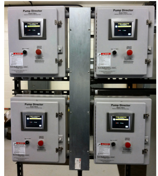
Each pump control valve has its own dedicated Model 7700A Pump Director. It can be installed near the valve it controls or at a more convenient location, as shown above for a (4) pump arrangement.
