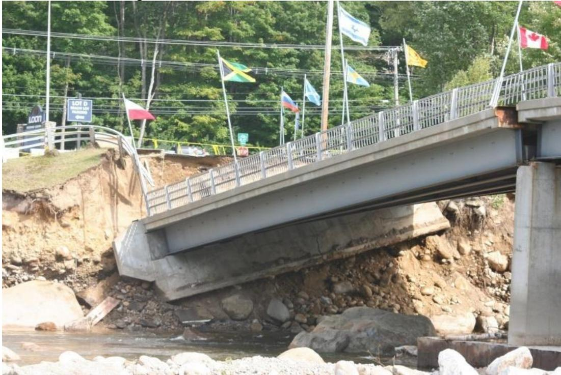
**Figure 4. Photo of the failed Loon Mountain Bridge abutment.**
