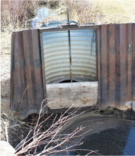
Headgate looking downstream
