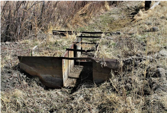
Flume looking downstream
