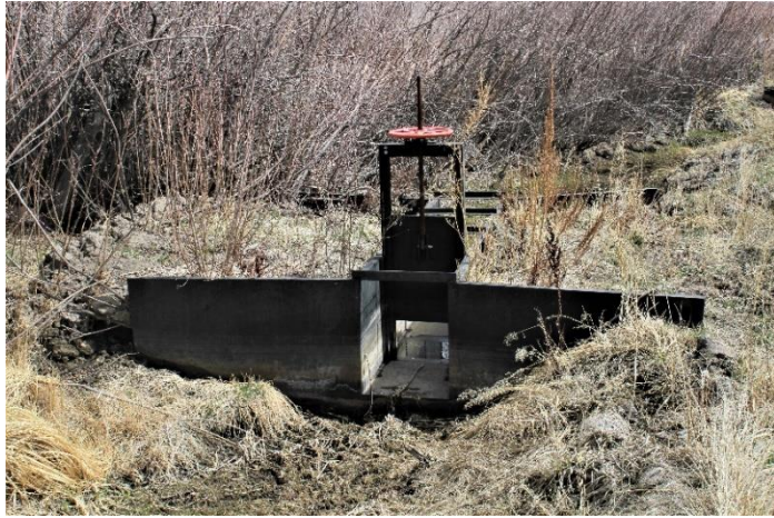
Headgate looking downstream
