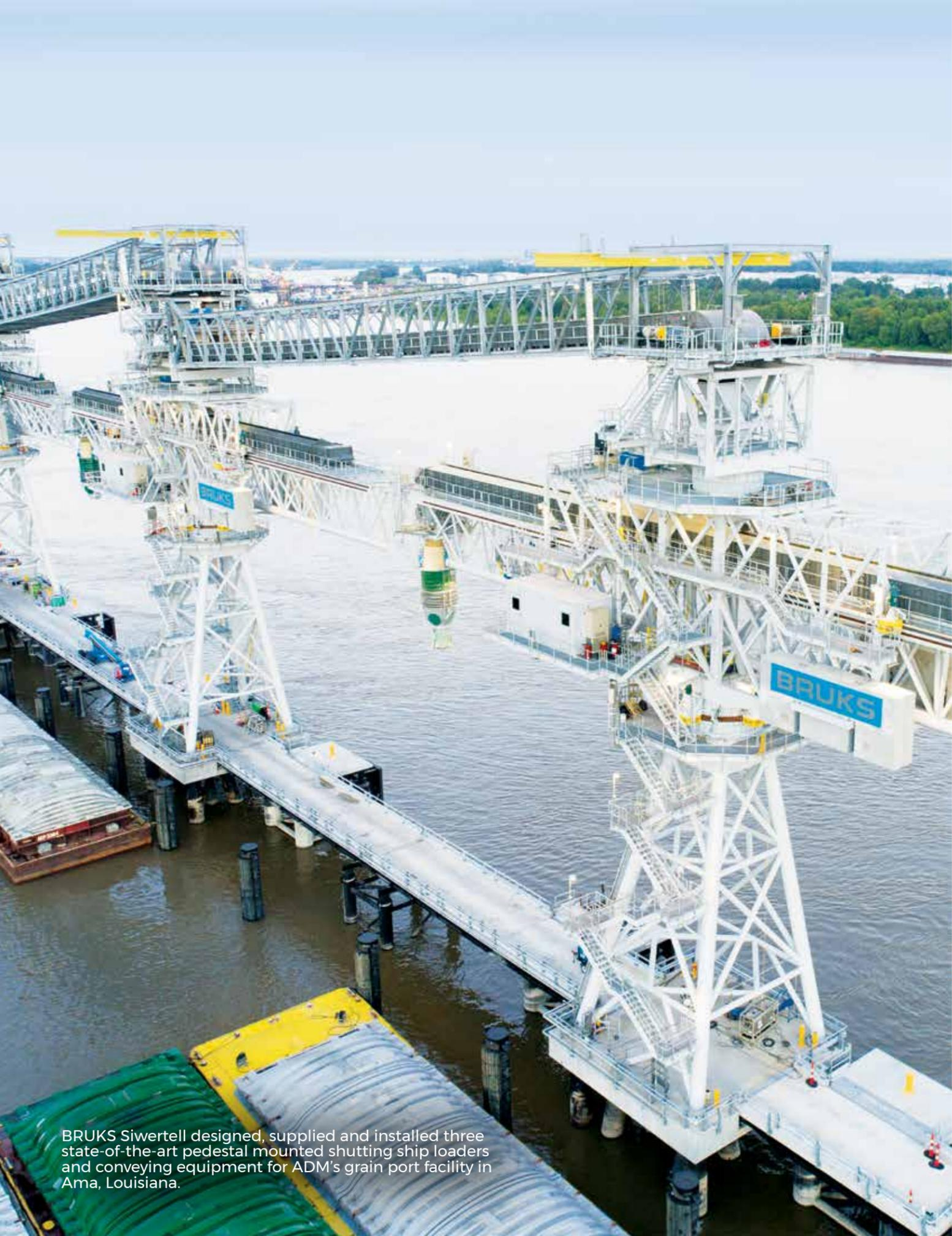
BRUKS Siwertell designed, supplied and installed three state-of-the-art pedestal mounted shutting ship loaders and conveying equipment for ADM's grain port facility in Ama, Louisiana.
