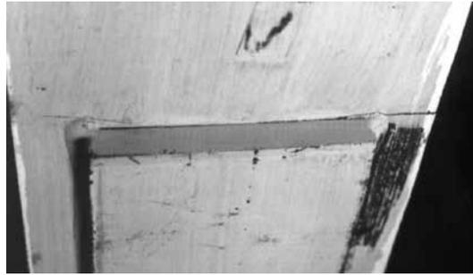
Figure 3. Fatigue crack at the end of a cover plate fillet weld toe (U.S. DOT, *Bridge Design Handbook, Design for Fatigue*).
