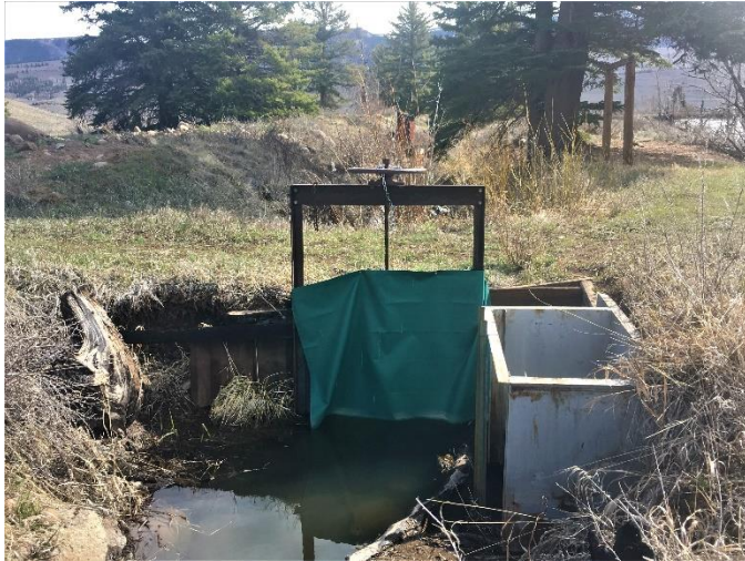
Headgate looking downstream
