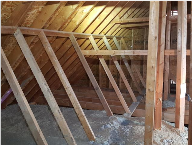
main attic area
