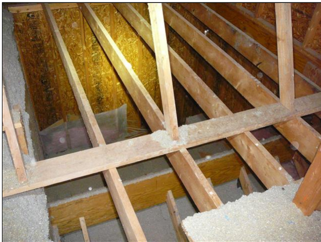
main attic area
