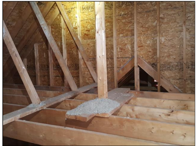
main attic area
