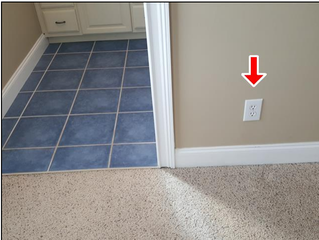
6.7 Item 3(Picture) 3rd bedroom
