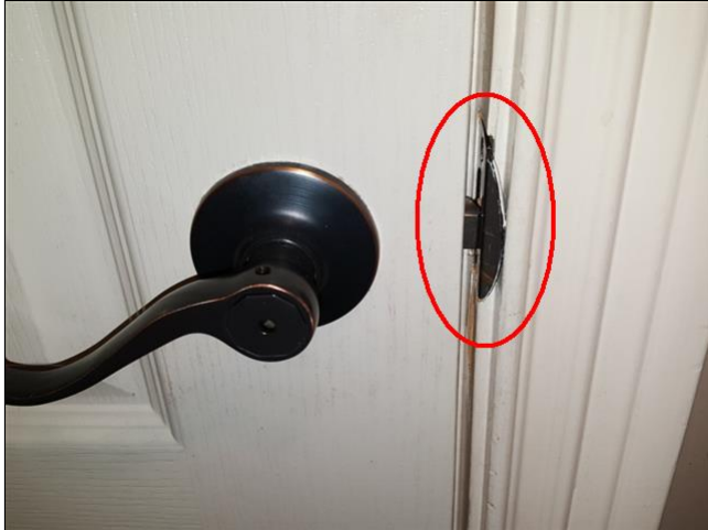
6.4 Item 5(Picture) washer dryer room
