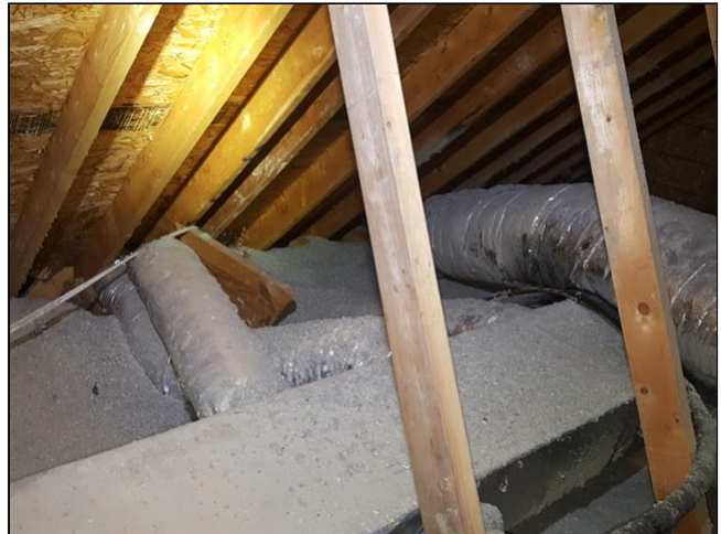
main attic area
