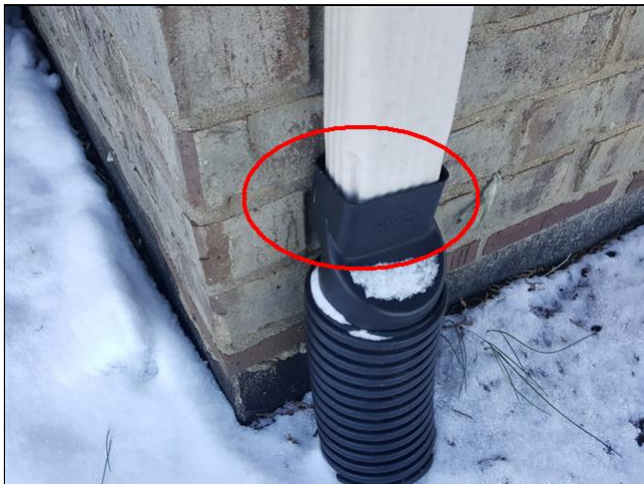
2.3 Item 9(Picture) front right corner of home
