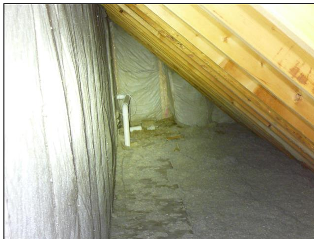
bonus room attic area
