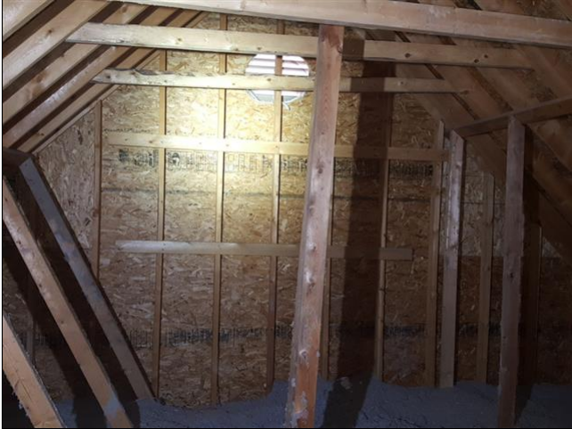
main attic area
