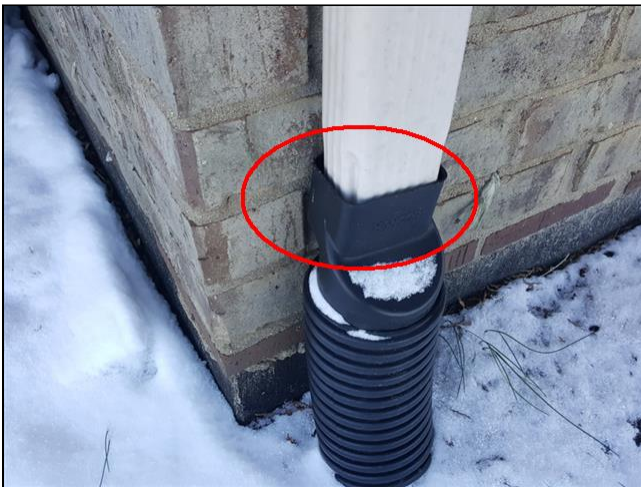
2.3 Item 9(Picture) front right corner of home
