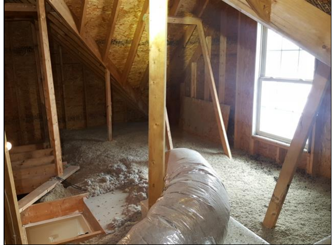
main attic area
