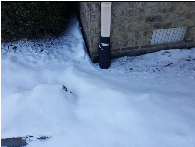
2.3 Item 5(Picture) front right corner of home
