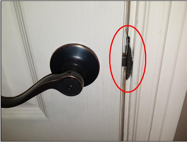
6.4 Item 5(Picture) washer dryer room
