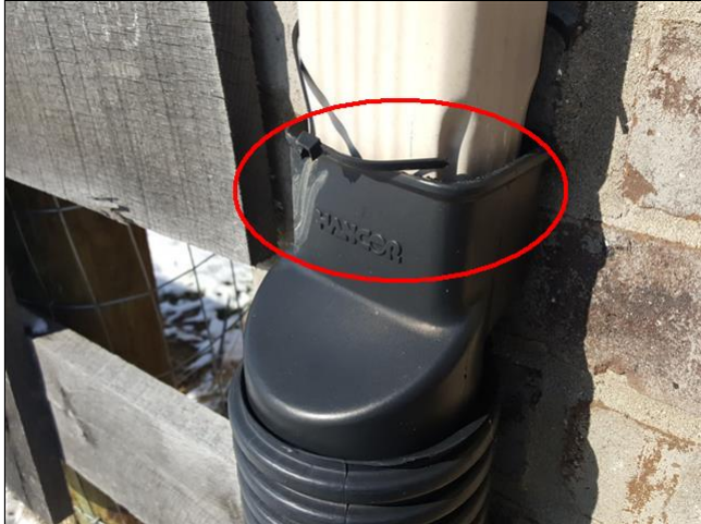
2.3 Item 7(Picture) rear right corner of home
