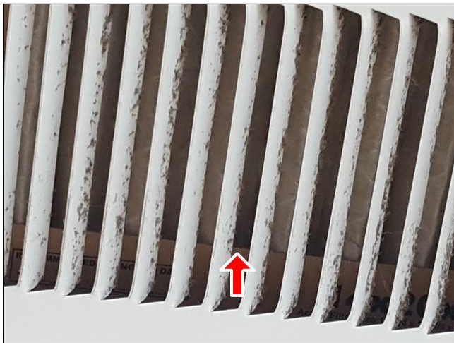
10.1.B Item 3(Picture) hallway ceiling upstairs
