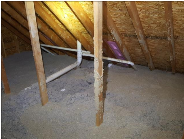
main attic area
