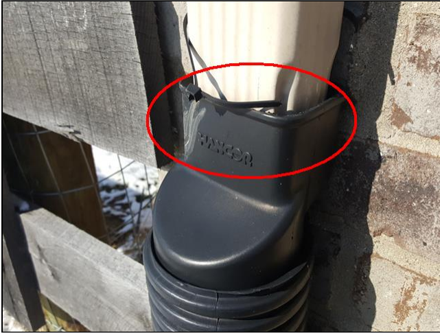
2.3 Item 7(Picture) rear right corner of home
