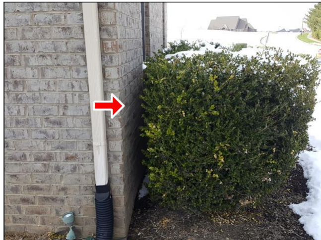
3.11 Item 3(Picture) side of garage
