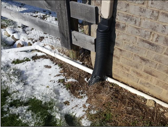
2.3 Item 3(Picture) rear right corner of home
