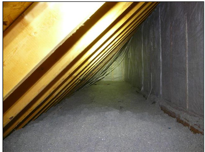
bonus room attic area
