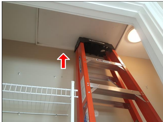
2.4 Item 2(Picture) 2nd bedroom closet
