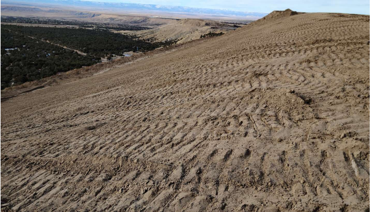
Face of Lift #4 – soil cover in process – photo looking northwest
