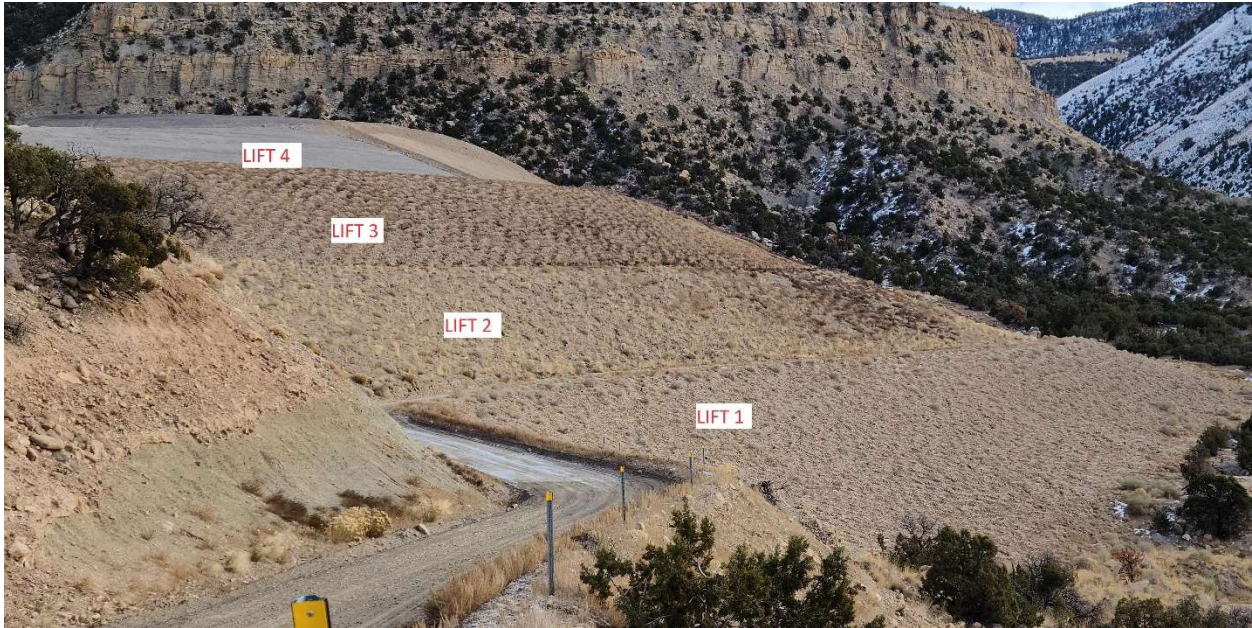
SCA#2 Ash Landfill –looking southeasterly
