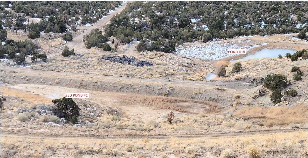
Sediment Trap #1 is empty and clean water flows from trap to pond 018 in normal open condition.
