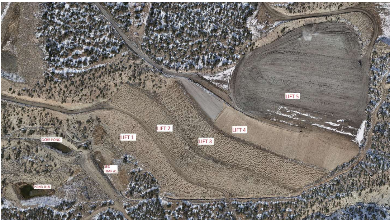
SCA#2 Ash Landfill – Aerial view Lift #5 in progress
