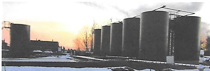
An injection well in Mayfield Township, Grand Traverse County.
