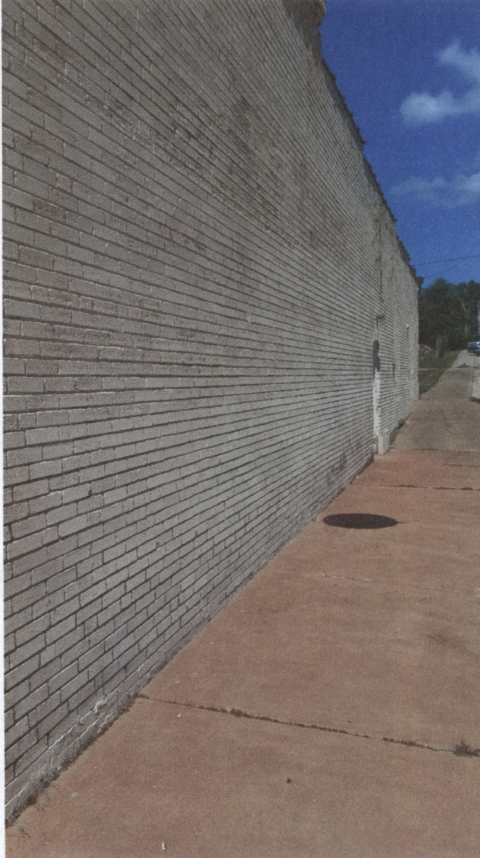
200 N. Lincoln Street – Exterior view the south side of the building.
