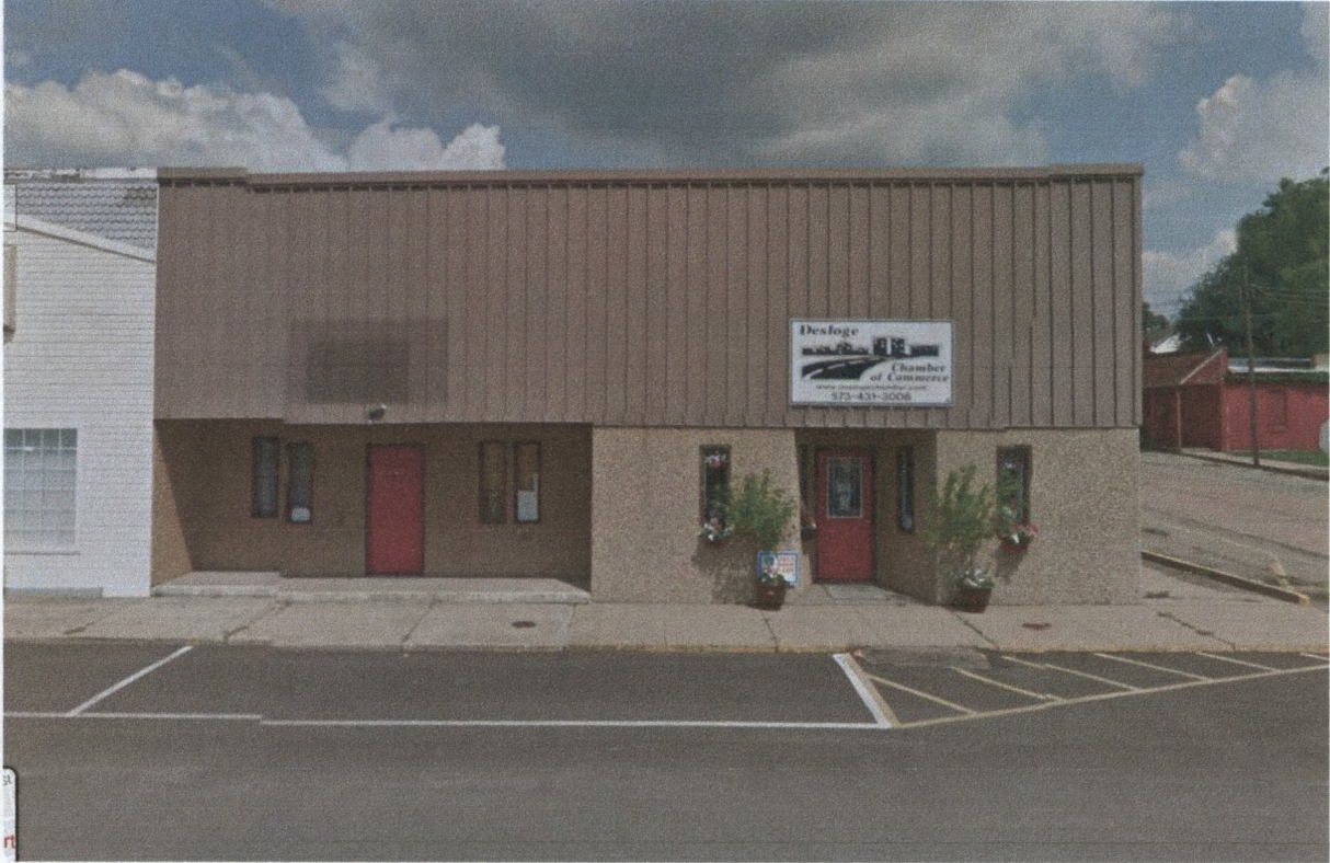
200 N. Lincoln Street – Front view of building.
