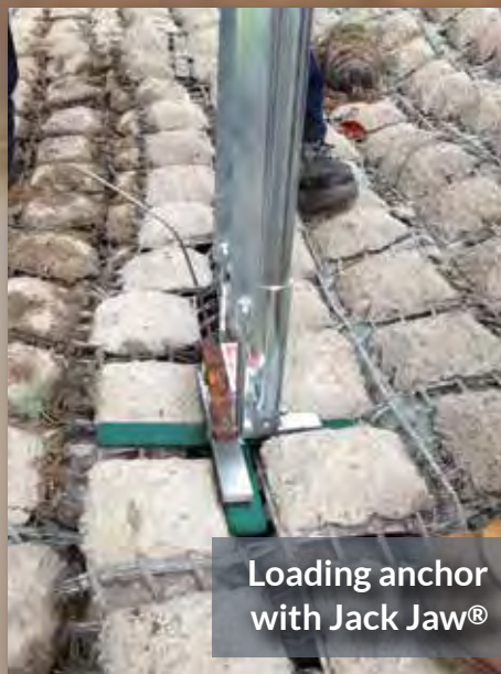
Gas powered driver installation
