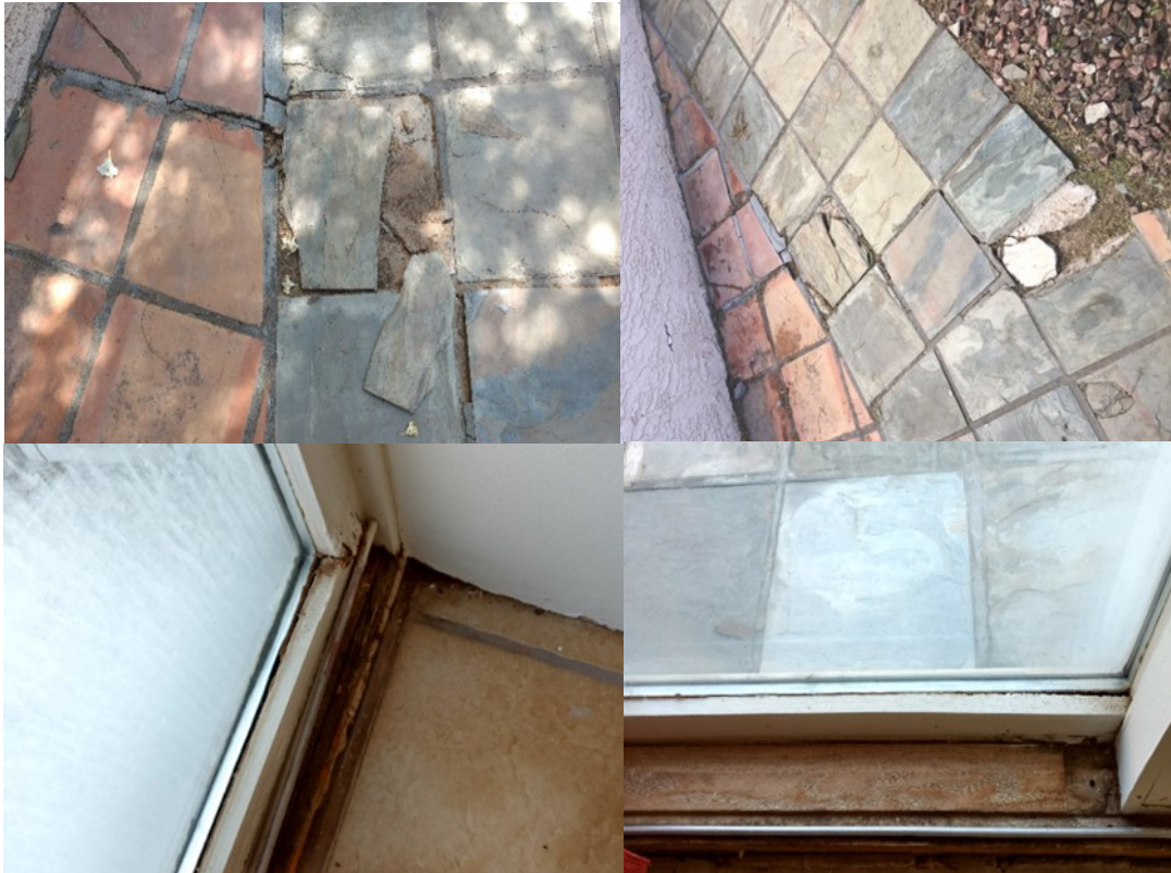
Broken tiles and damaged door frame
