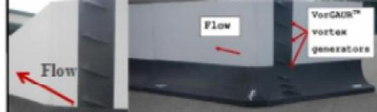
**Example stainless steel scAUR™ retrofit (black) for a 45° wing-wall abutment. Note SS vortex generators.**
