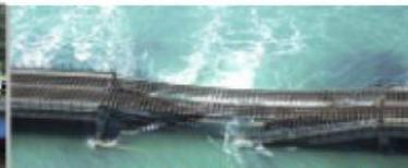
**Scour caused Irish railway bridge pier collapse minutes after passage of a full Dublin-to-Belfast commuter train, 3 September 2009.**
