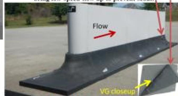
Example stainless steel scAUR™ retrofit (black) for a 45° wing-wall abutment. Note SS vortex generators.
