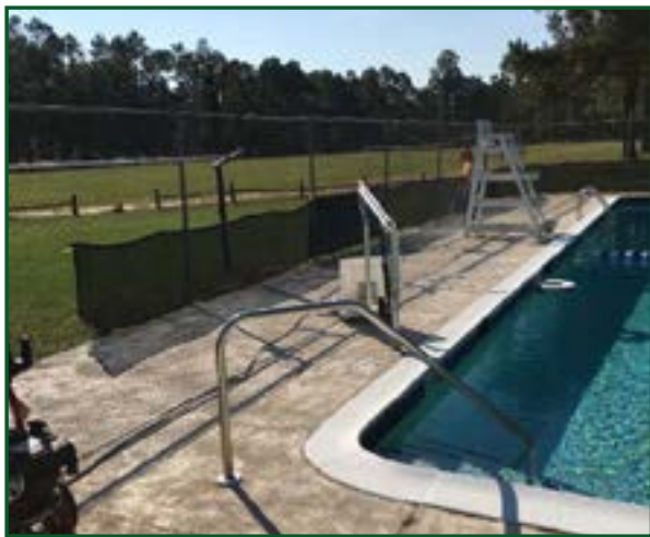
Pool deck repair
