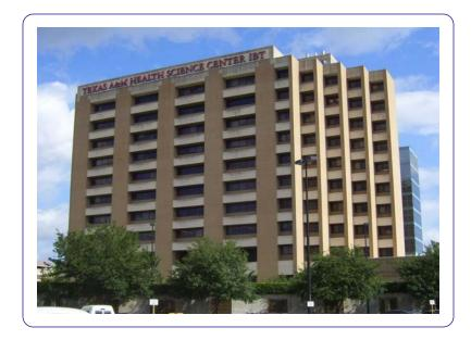
The IBT is an eleven-story concrete frame office building and an adjacent two-story laboratory wing constructed around 1989. The exterior walls are constructed with brick masonry veneer and CMU backup walls, precast concrete spandrel beams and sunscreens, and aluminum framed windows.
