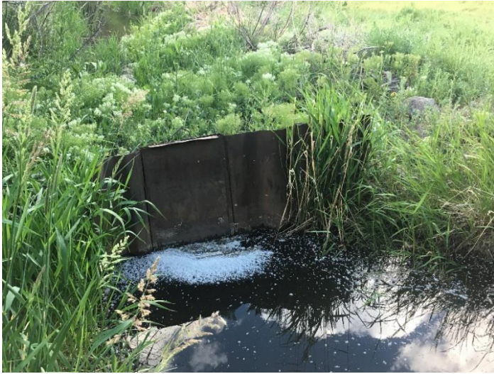
Headgate looking downstream
