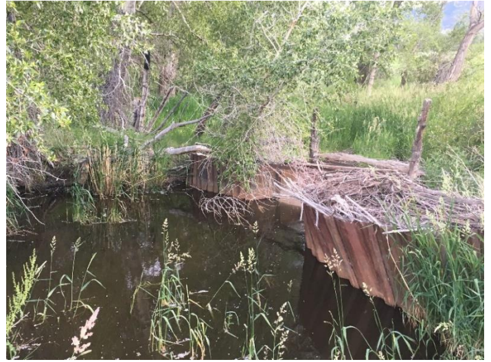
Diversion dam looking downstream
