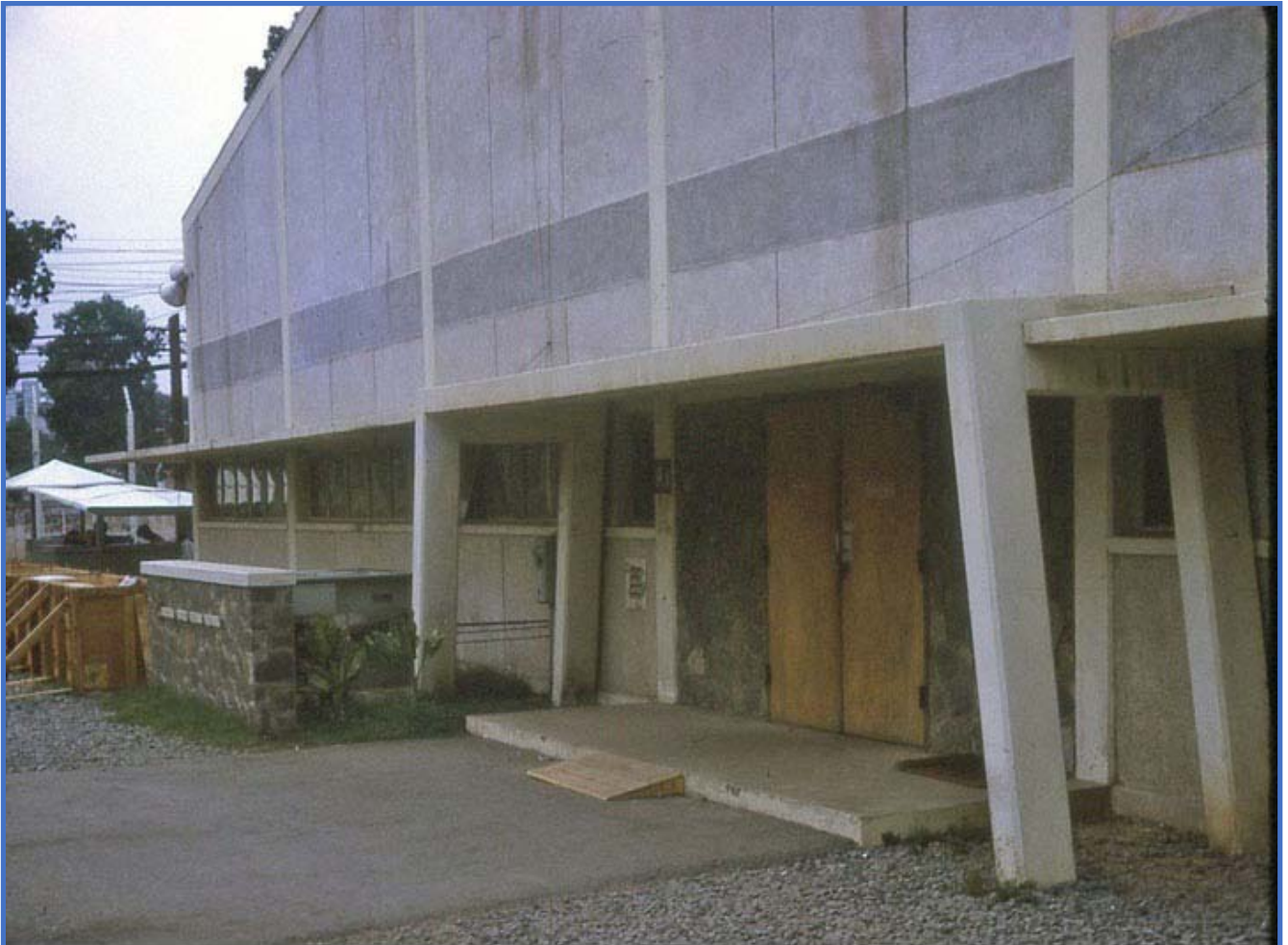
The front entrance. Note the additional barricade near the guard station.
