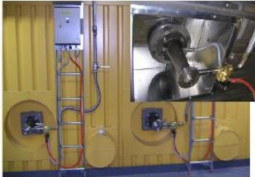
**Acoustic gas temperature measurement system**
