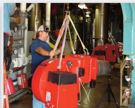
Step 4. Install new Weishaupt high efficiency burner assembly.
