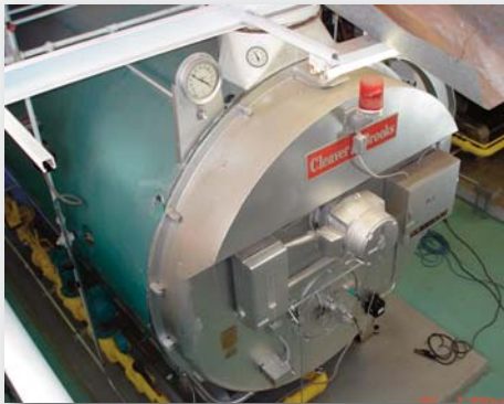
Cleaver Brooks Fire Tube Boiler
