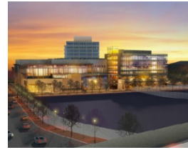
Tysons West JBG Rosenfeld Phase I includes a Walmart that opened in 2013. Will have 1.3 MSF at total build out
