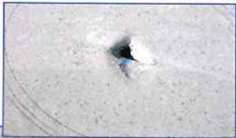
Right: Photo 4 – Large puncture in single-ply membrane.
