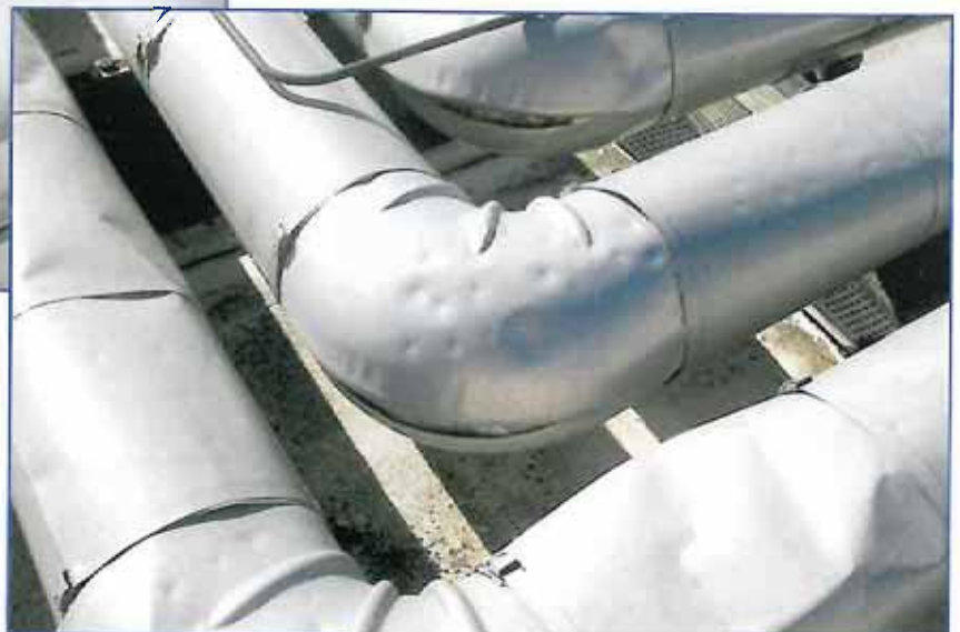
Photo 19: Dents in metal jacket on insulated piping.
