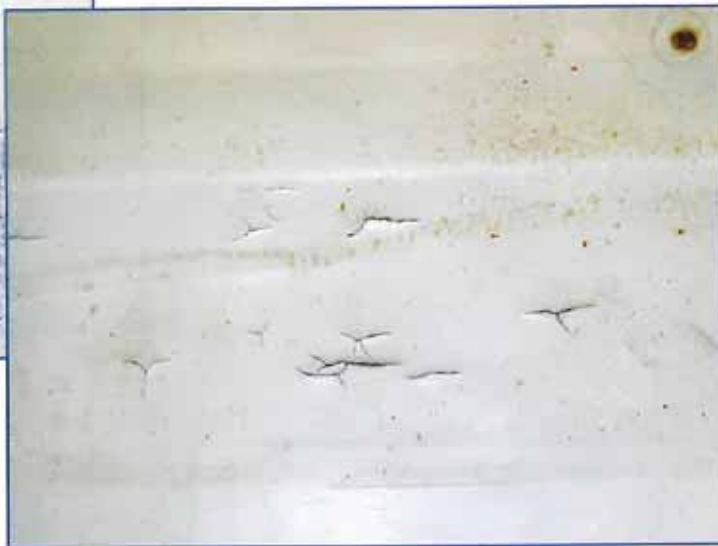
Photo 33 - View of damage on bottom of membrane.
