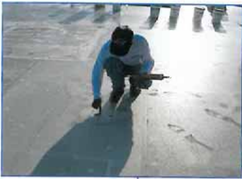
Photo 24 – Applying sealant to damaged areas on single-ply.
