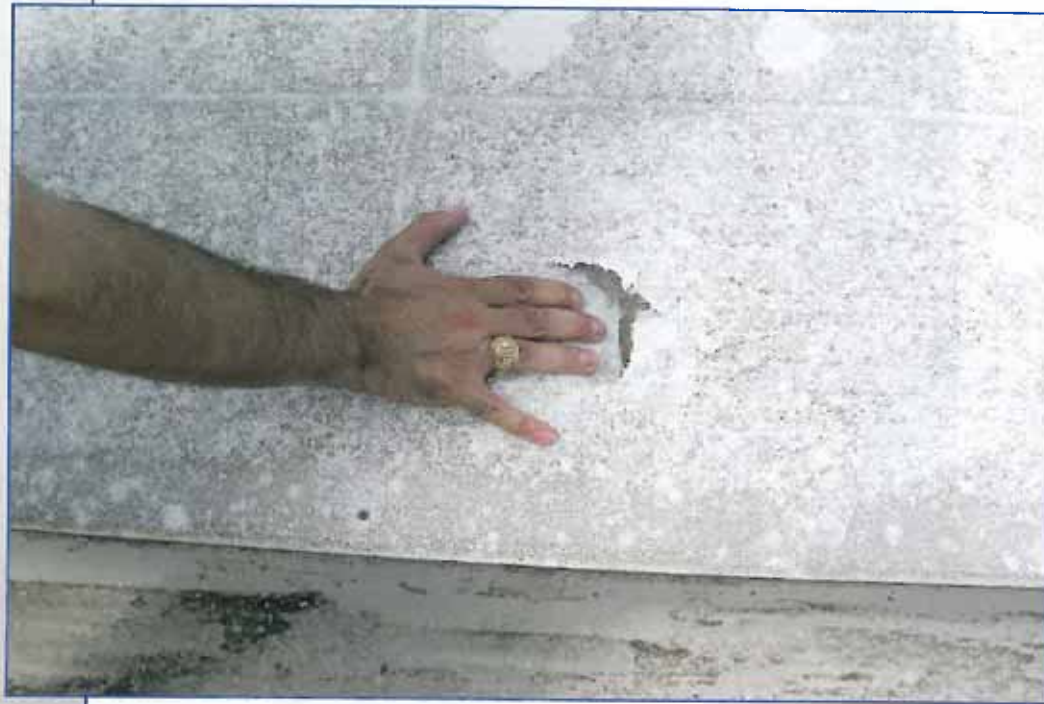
Photo 17 – Puncture in fabric skylight.
