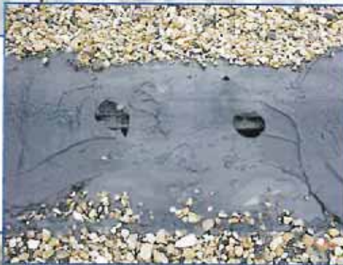
Photo 9 – Punctures in weathered expansion joint.
