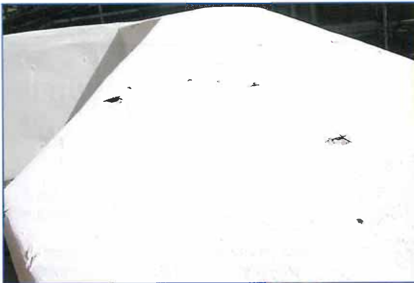
Photo 22 – Punctures in exterior insulated duct.
