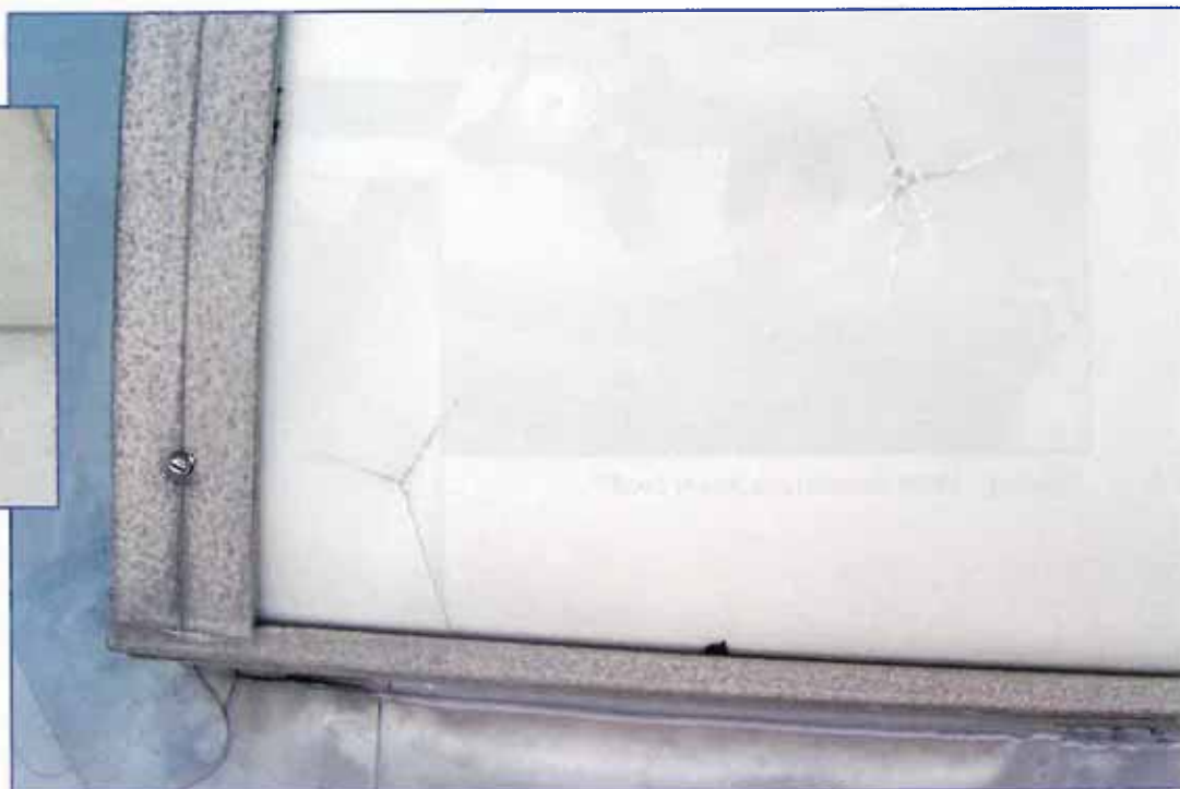
Photo 14 – Fracture in fiberglass skylight.
