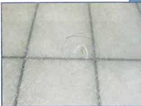
Photo 14 – Fracture in fiberglass skylight.
