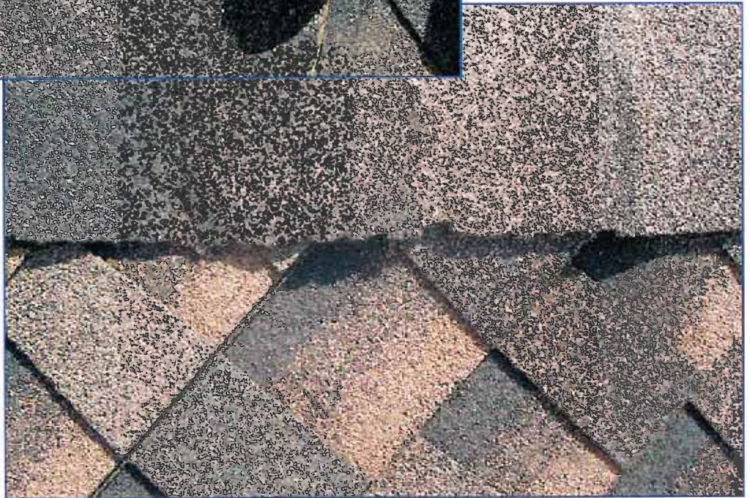
Photo 13 – Damage to edges of ridge shingles.
