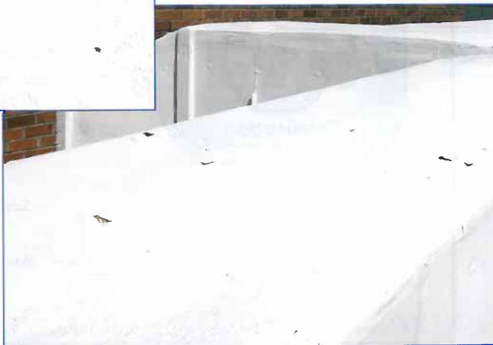
Photo 23 – Punctures in exterior insulated duct.
