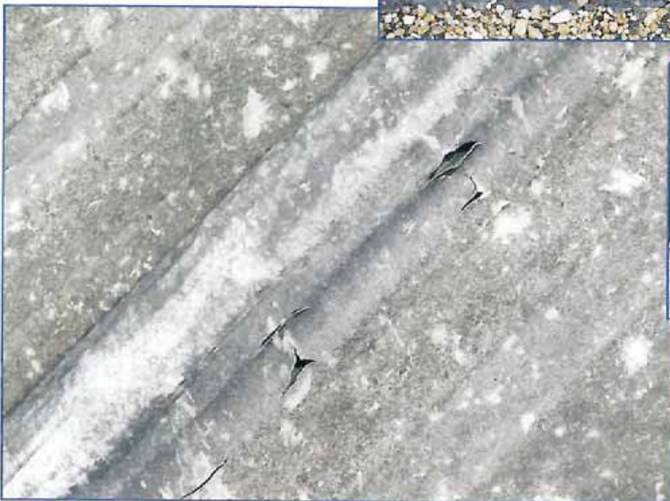
Photo 11 – Large dents in metal canopy.
