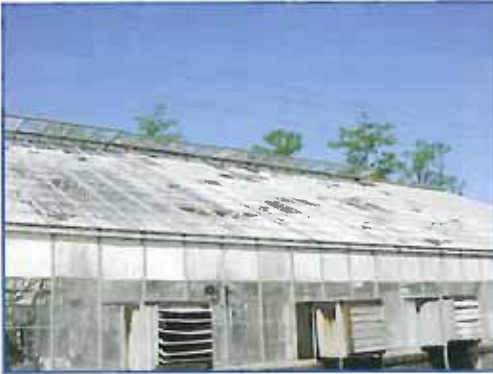
Photo 21 – Significant damage to glass panels.
