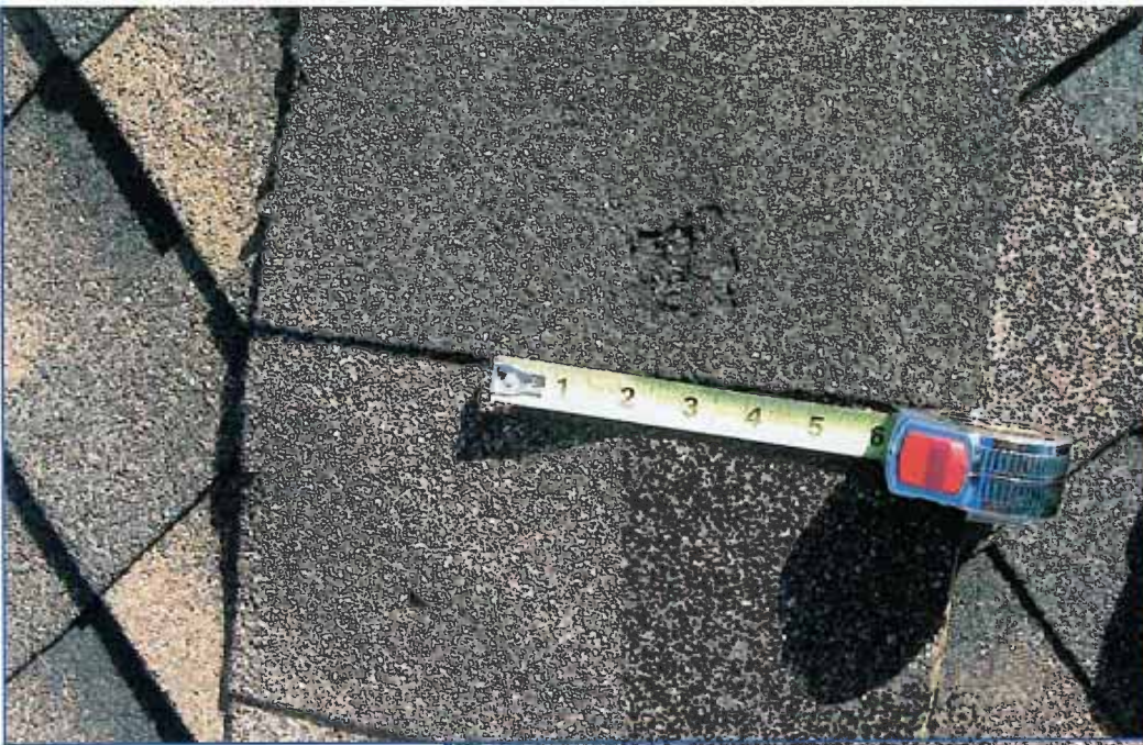
Photo 12 – Large impact on ridge shingle.
