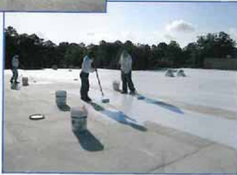
Photo 25 – Applying coating to damaged single-ply membrane.
