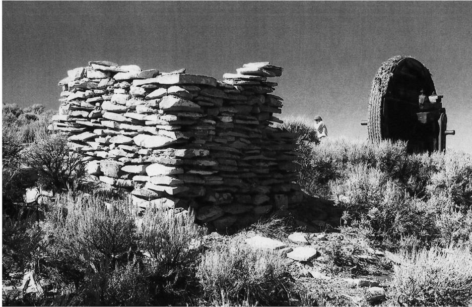
Figure 13: Stone platform possibly to support a steam boiler with a bull wheel shown in the background between the McNaughton #9 and #10 wells.
