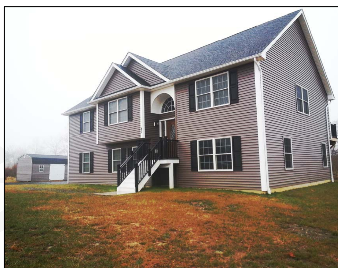
viewed looking southeasterly
