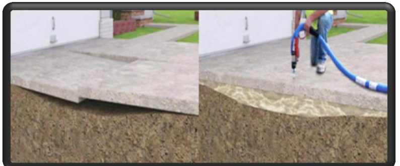
Example of a successful repair
