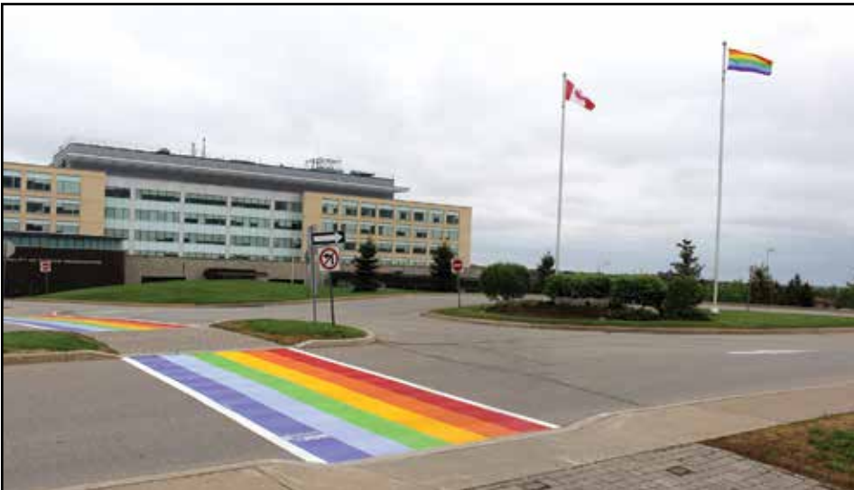
The Region of Durham is sending a message of inclusion to everyone who visits its corporate headquarters building in Whitby, with the installation of a new rainbow crosswalk, just in time to kick off Pride Month in Durham Region. Durham Region's rainbow crosswalk was installed in-house by Works Department staff.
