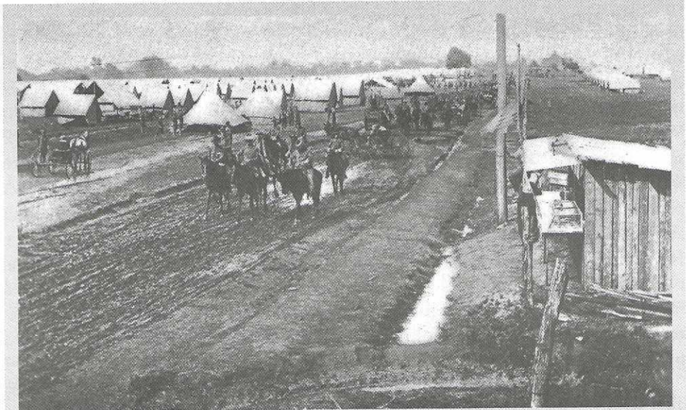
Volunteers' Encampment along Charlottesville Road (Rte 231)
