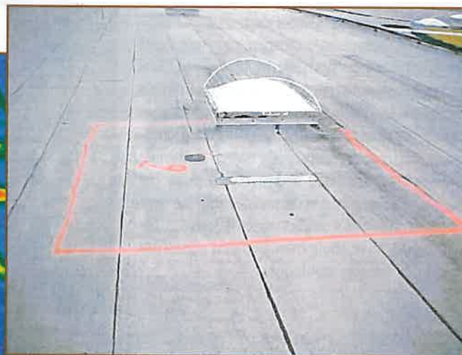
Photograph 6: View of anomaly of wet ISO under modified-bitumen membrane.
