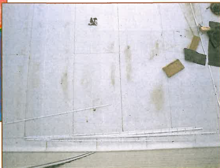
Photo 11 – View of soiled areas of white-surfaced modified-bitumen cap sheet.
