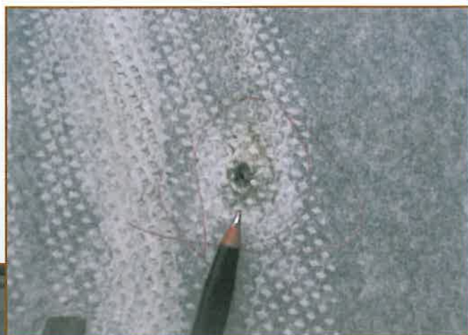
Photo 9 – Small hole in membrane that was source of water entry.
