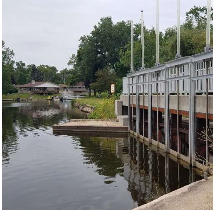
2019 View of Embankment Wall
