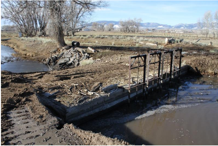
Headgate looking downstream
