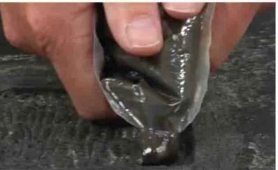
Cut open any corner of the resin pack and squeeze out the resin on to the damaged surface area.
