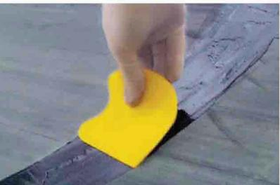
Smooth the resin to the desired level using a flat edged putty knife or Eli-Flex spatula (available on request). Leave to cure (see below curing times).
