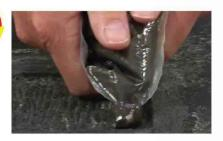
Cut open any corner of the resin pack and squeeze out the resin on to the damaged surface area.
