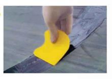
Smooth the resin to the desired level using a flat edged putty knife or Eli-Flex spatula (available on request). Leave to cure (see below curing times).
