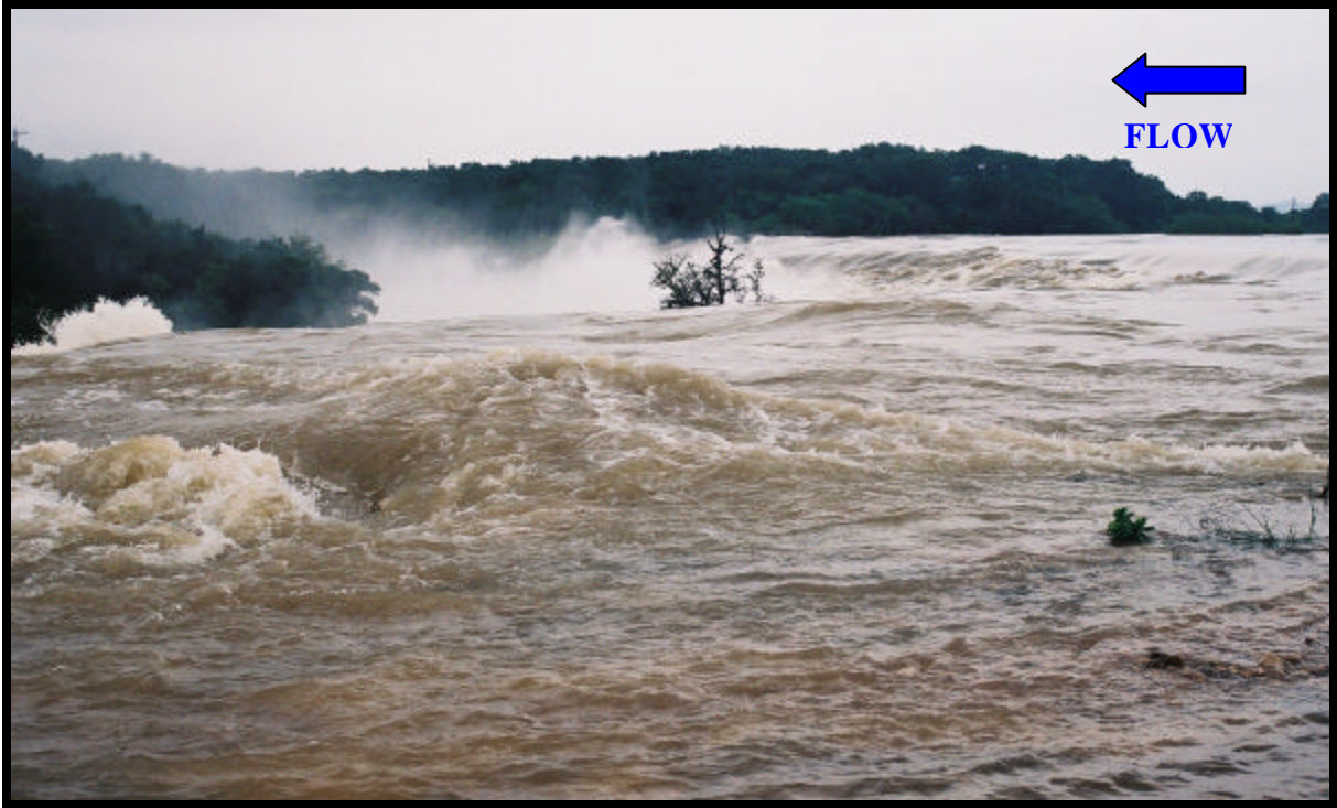
Photo 16 View of discharge over emergency spillway, looking upstream from the right abutment. Note the turbulent flow and standing waves approaching the spillway “lip”. (Friday, July 5 th )
