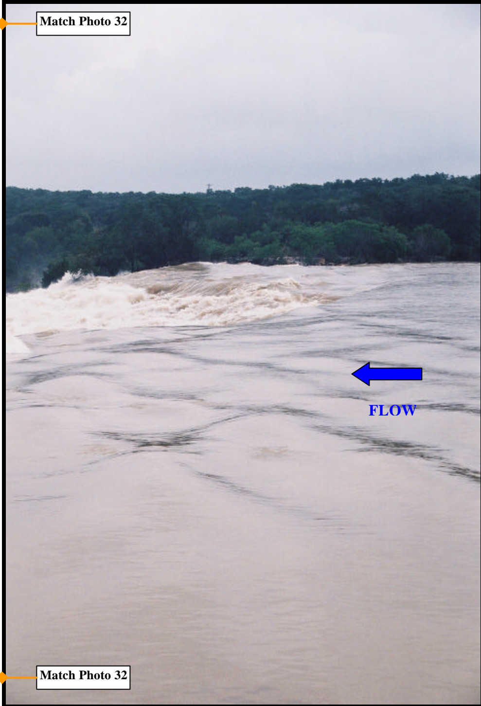
Photo 33 Panoramic view of emergency spillway, looking right. (Saturday, July 6 th )
