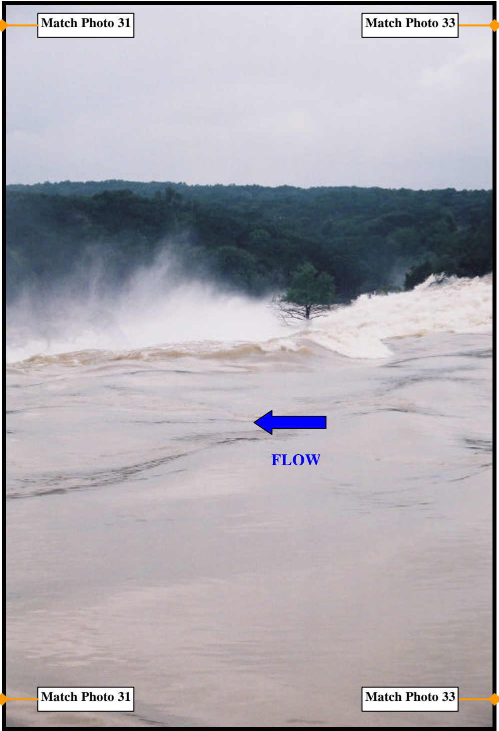
Photo 32 Panoramic view of emergency spillway, looking right. (Saturday, July 6 th )
