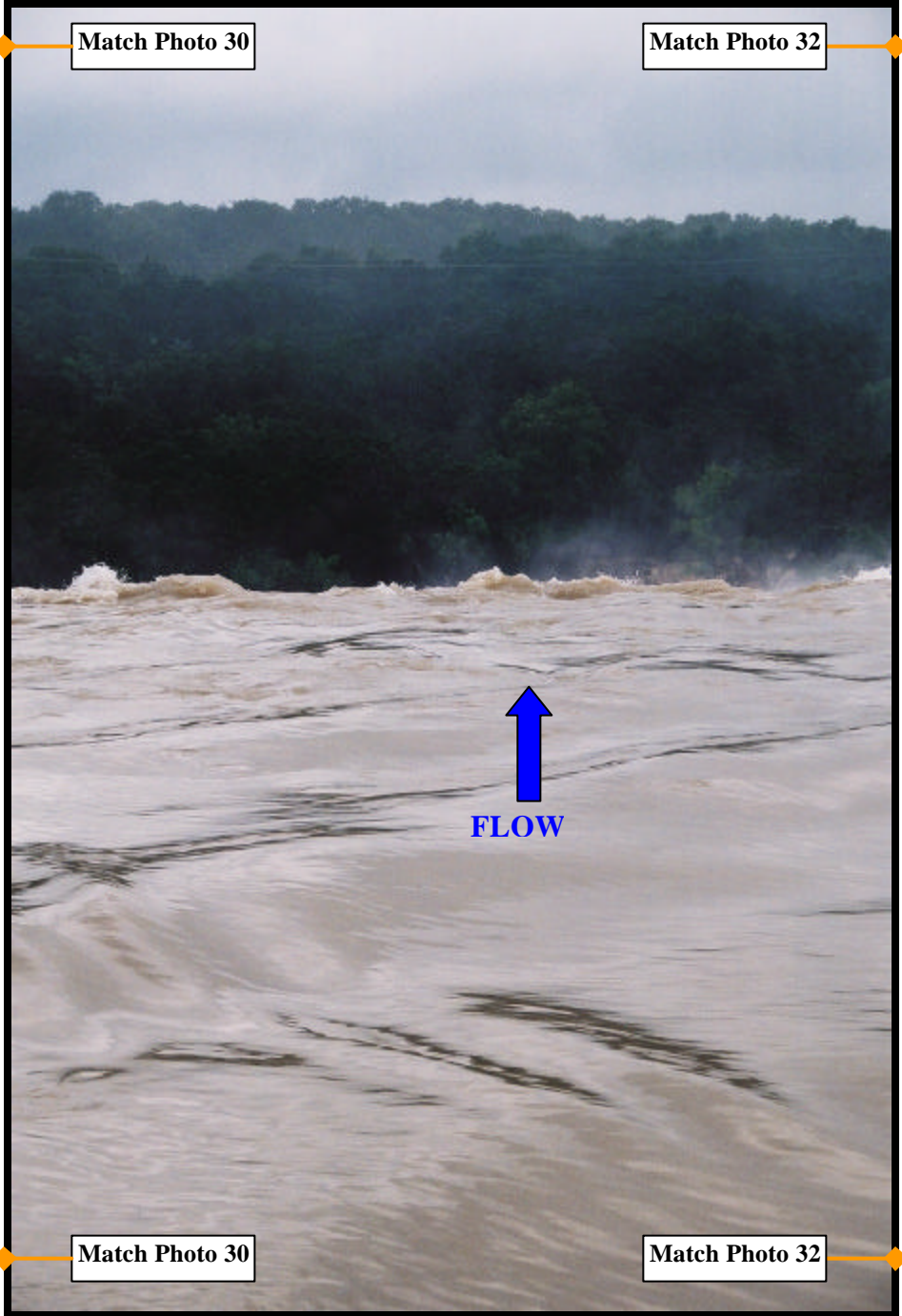
Photo 31 Panoramic view of emergency spillway, looking right. (Saturday, July 6 th )
