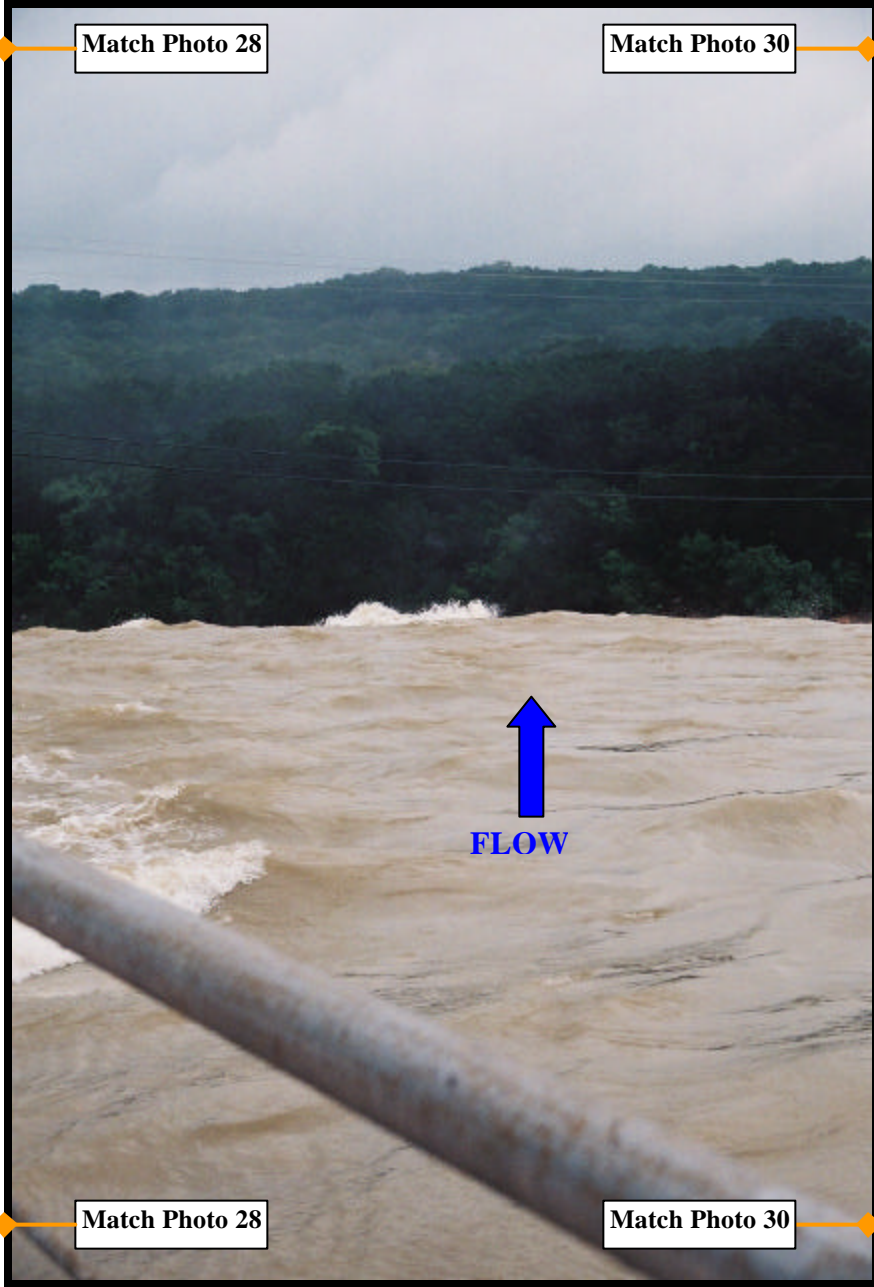
Photo 29 Panoramic view of emergency spillway, looking right. (Saturday, July 6 th )
