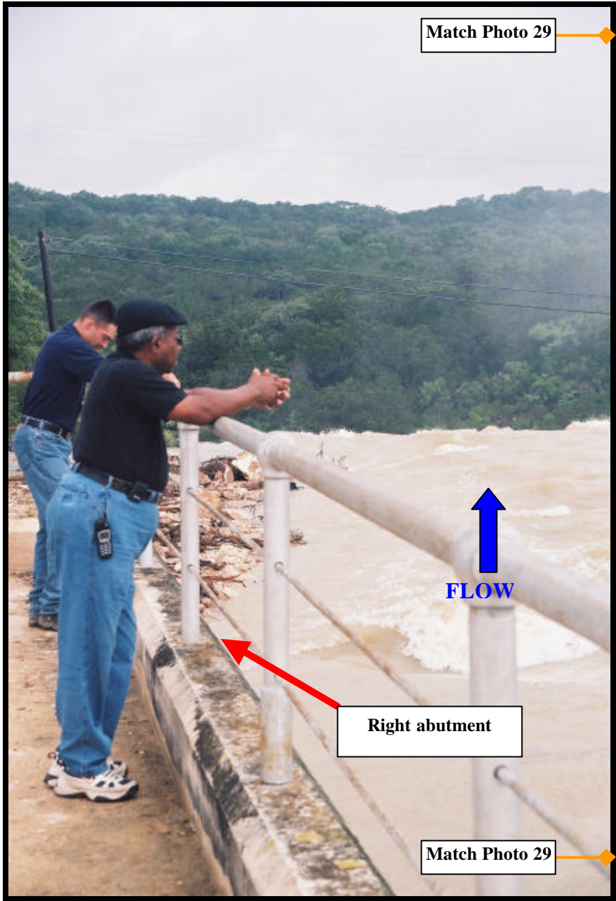
Photo 28 Panoramic view of emergency spillway, looking right. (Saturday, July 6 th )
