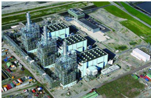
Vattenfall's Magnum power plant in the Netherlands is shown here. Mitsubishi Hitachi Power Systems (MHPS) has verified that conversion to hydrogen-fired power generation is possible on these units. Photo courtesy: MHPS
