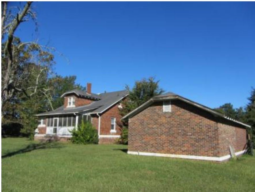
Figure 61. NCDOT Survey #15, Edwards House (GF-8177), 7210 Burlington Road, Guilford County, view of house and garage in foreground, looking northwest.
