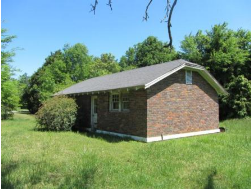
Figure 60. NCDOT Survey #15, Edwards House (GF-8177), 7210 Burlington Road, Guilford County, garage, southwest corner, looking northeast.
