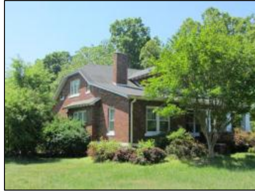
NCDOT Survey #15, Edwards House (GF-8177), 7210 Burlington Road, looking southwest.
