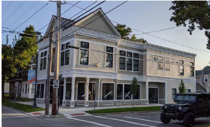
Figure 1015. This new building exemplifies many desired design elements including facade breaks, use of traditional windows, short setbacks to the street, and traditional siding. This building could house commercial on the ground floor, and commercial and/or residential on the second floor.
