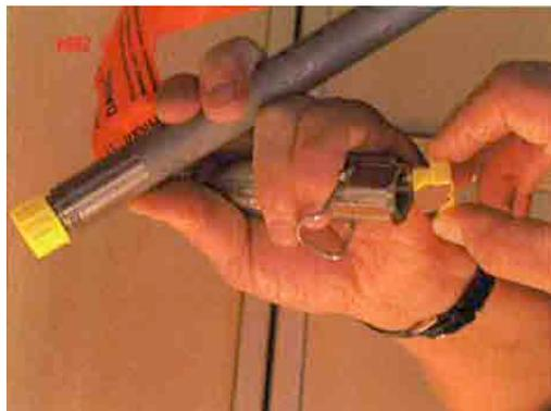
**Figure 11** Putting on protective plastic cap and plug.
