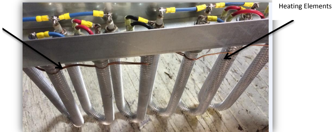
Figure 10 Reheat Elements
