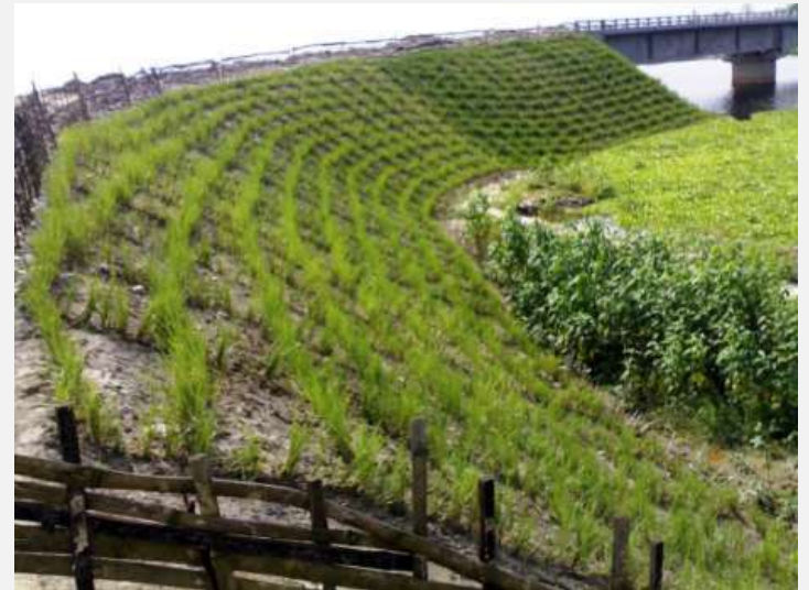
Bridge abutment, Assam,
