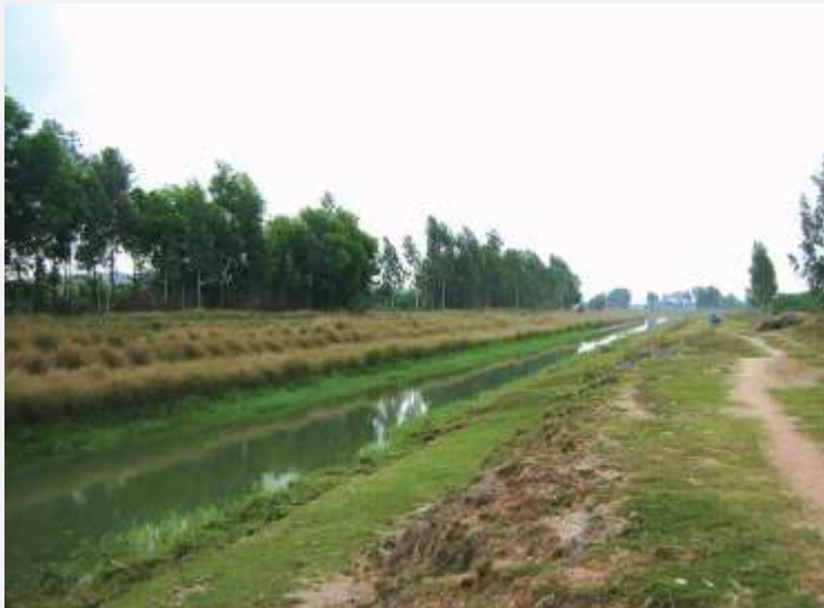
Canal and storm dike protection (Vietnam); India
