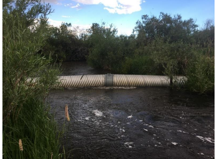
Pipeline across Saguache Creek
