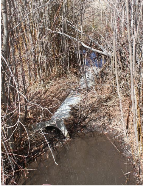
Culvert looking downstream
