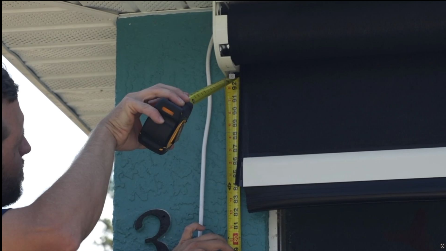
Measuring tacks before cutting tracks
