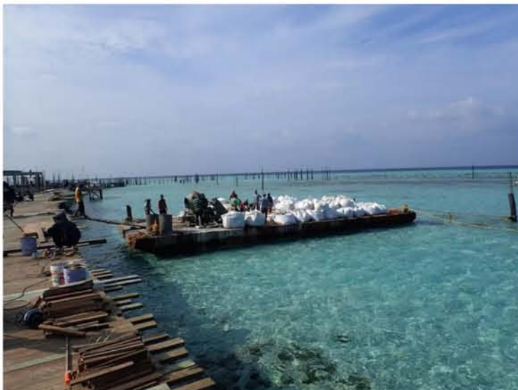
A resort construction site – a regular sight now in the Maldives
