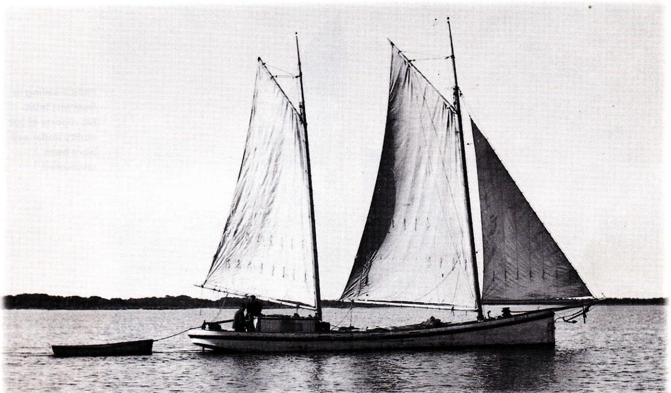
BESSIE D ghosts along in what, to date, is the only known photograph of a sharpie rigged as a "yallowicker," an apparently whimsical name used colloquially for this ketch-like rig, characterized by the absence of standing rigging and spring stay.
