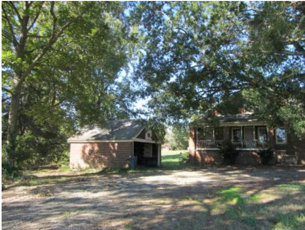
Figure 85. NCDOT Survey #12, Ingle House (GF-8174), 7232 Burlington Road, Guilford County, view of garage and east elevation of main house, looking west-northwest.
