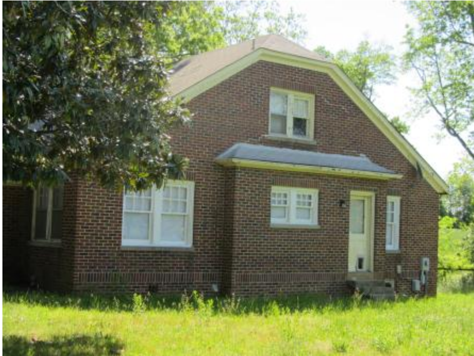
Figure 84. NCDOT Survey #12, Ingle House (GF-8174), 7232 Burlington Road, Guilford County, rear (south) elevation, looking northeast.
