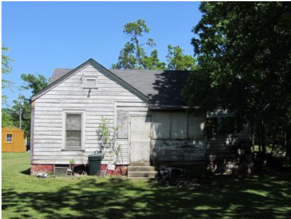
Figure 94. NCDOT Survey #16, Gaither House (GF-8178), 7206 Burlington Road, Guilford County, south elevation, looking north, with portable sheds visible on the left.
