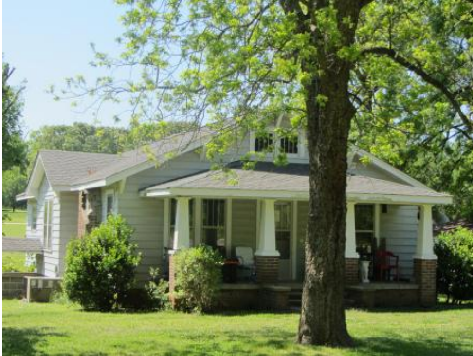
Figure 87. NCDOT Survey #13, Friddle House (GF-8175), 7226 Burlington Road, Guilford County, north façade, looking south.
